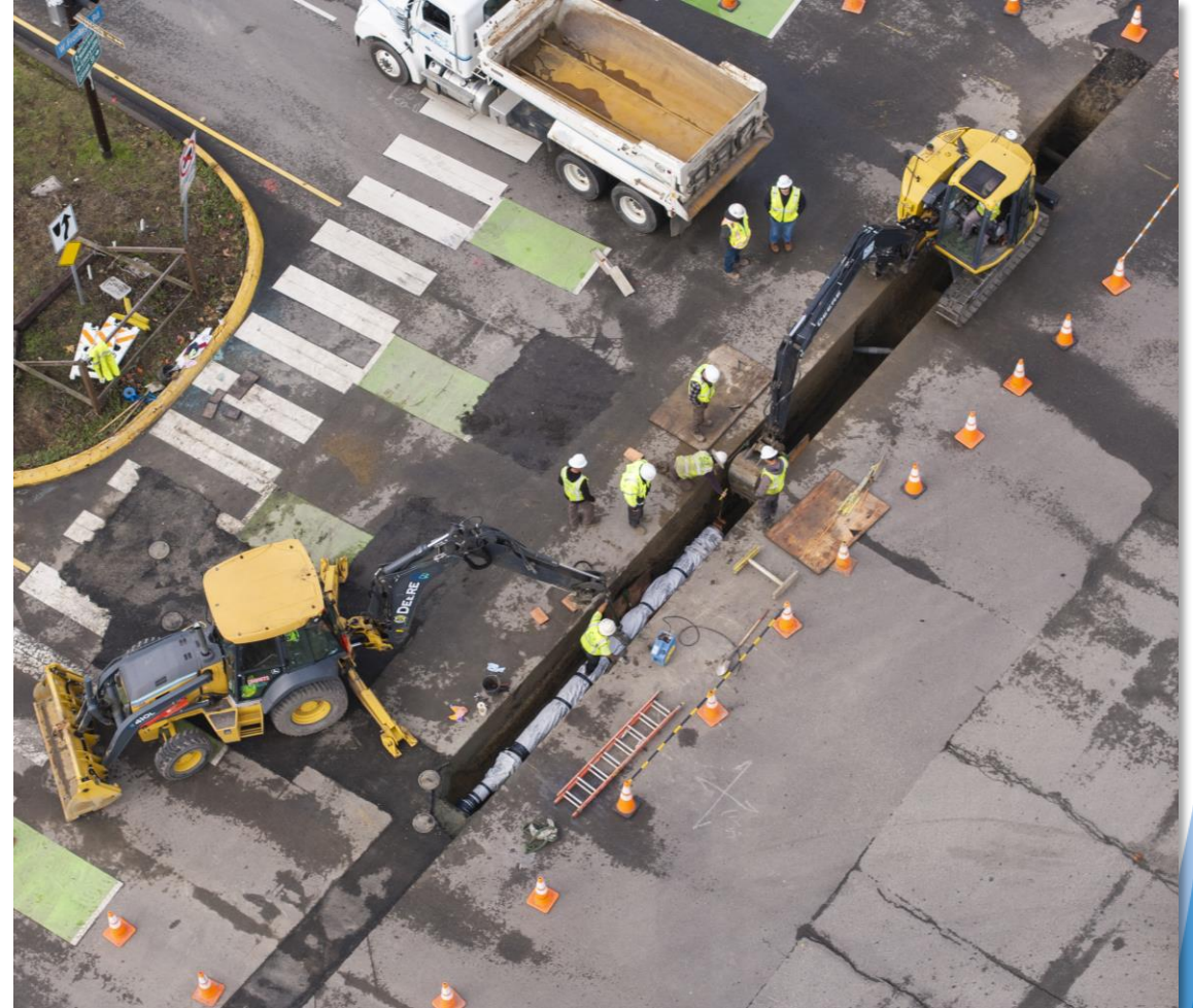
Frontage Rd pipeline installation, Berkeley, 2024
