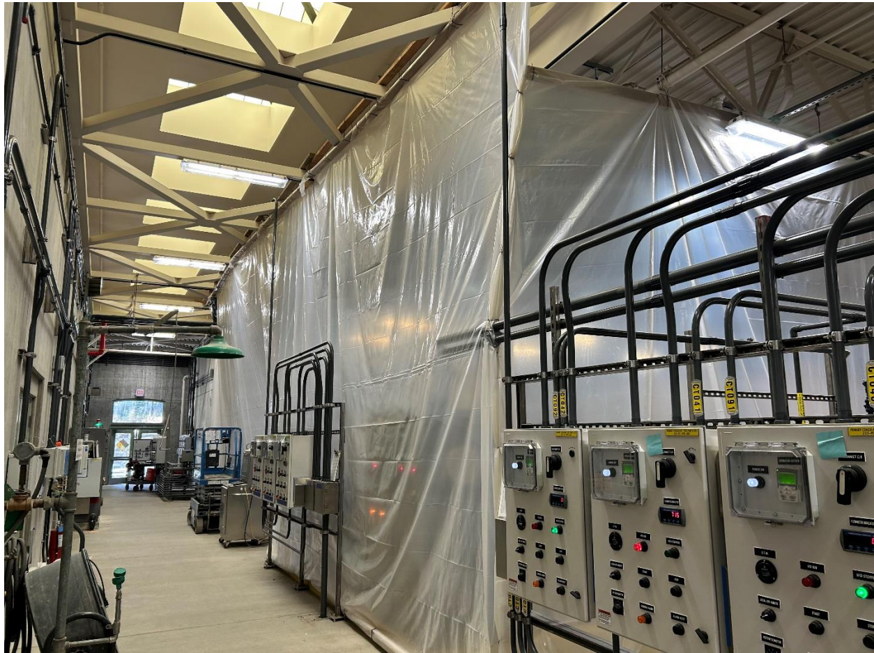
Photo 32 – Barrier wall installed in the Chemical Building to protect existing operations from dust and debris during demolition of old caustic soda systems as part of the Chemical Safety Systems Improvements portion of the project.
