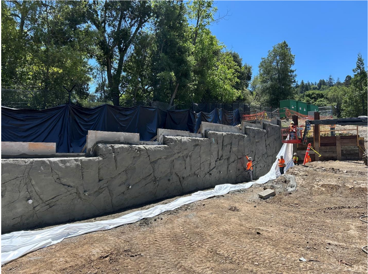
Photo 2 – Masons covering the fresh architectural finish on the shotcrete wall with plastic for curing. The completed retaining wall will support the hillside and allow for the installation of a foundation for the future South Electrical Building (SEB).
