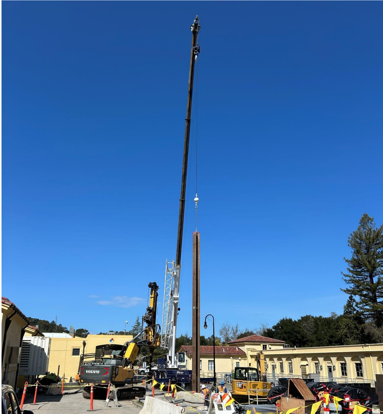
Photo 26 –A crane placing a steel beam to support the construction of a new chemical sump.
