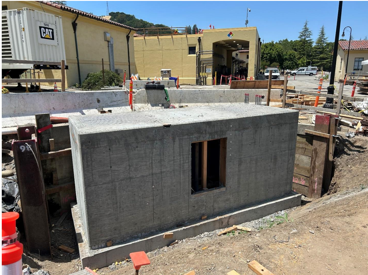
Photo 29 – Newly formed reinforced concrete chemical sump.
