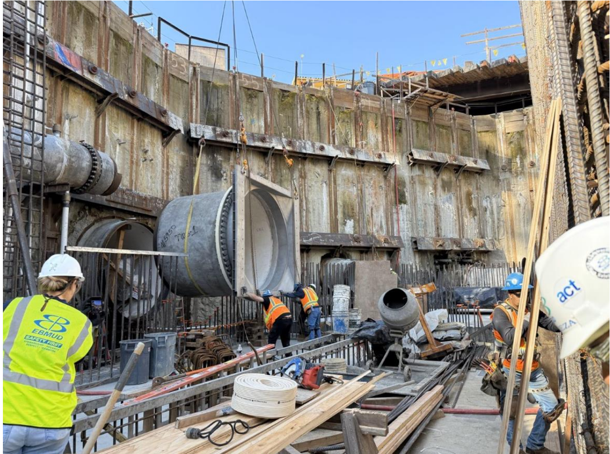
Photo 10 – Pipefitters pushing the 108-inch piping and wall gate thimble into place within the UV-CCB Facility with the aid of the tower crane.
