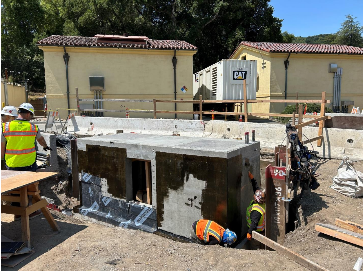
Photo 30 – Laborers applying waterproofing to new chemical sump 2 prior to backfill.
