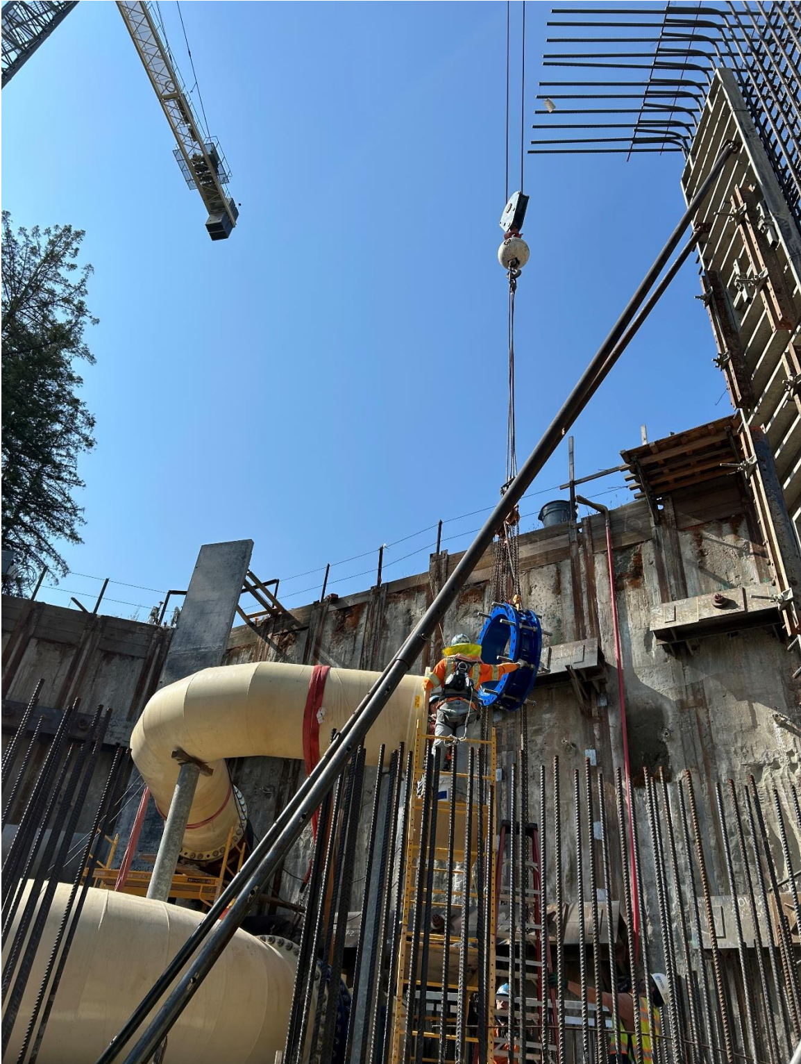
Photo 14 – Pipefitter positioning a flexible coupling on the 36-inch wasteway piping within the valve vault of the UV-CCB Facility with the aid of the crane.
