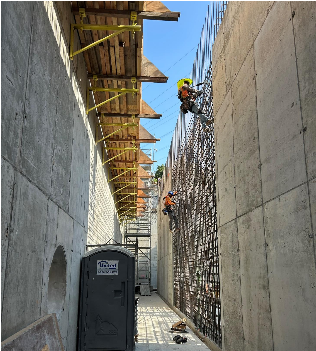
Photo 19 – Ironworkers tying rebar for the second level CCB wall. The first level of the CCB is located below the concrete floor in the photo. The round portal in the left wall is the piping for water entering the CCB from the adjacent UV Room.
