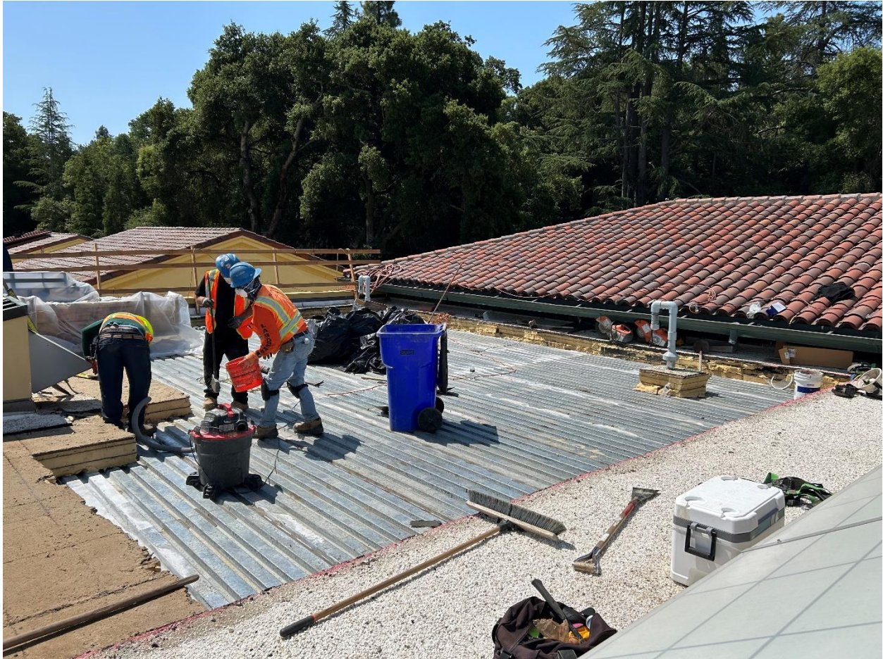
Photo 33 – Laborers performing selective demolition of the roofing system to install new skylights for the fluoride and ammonia rooms in the Chemical Building.
