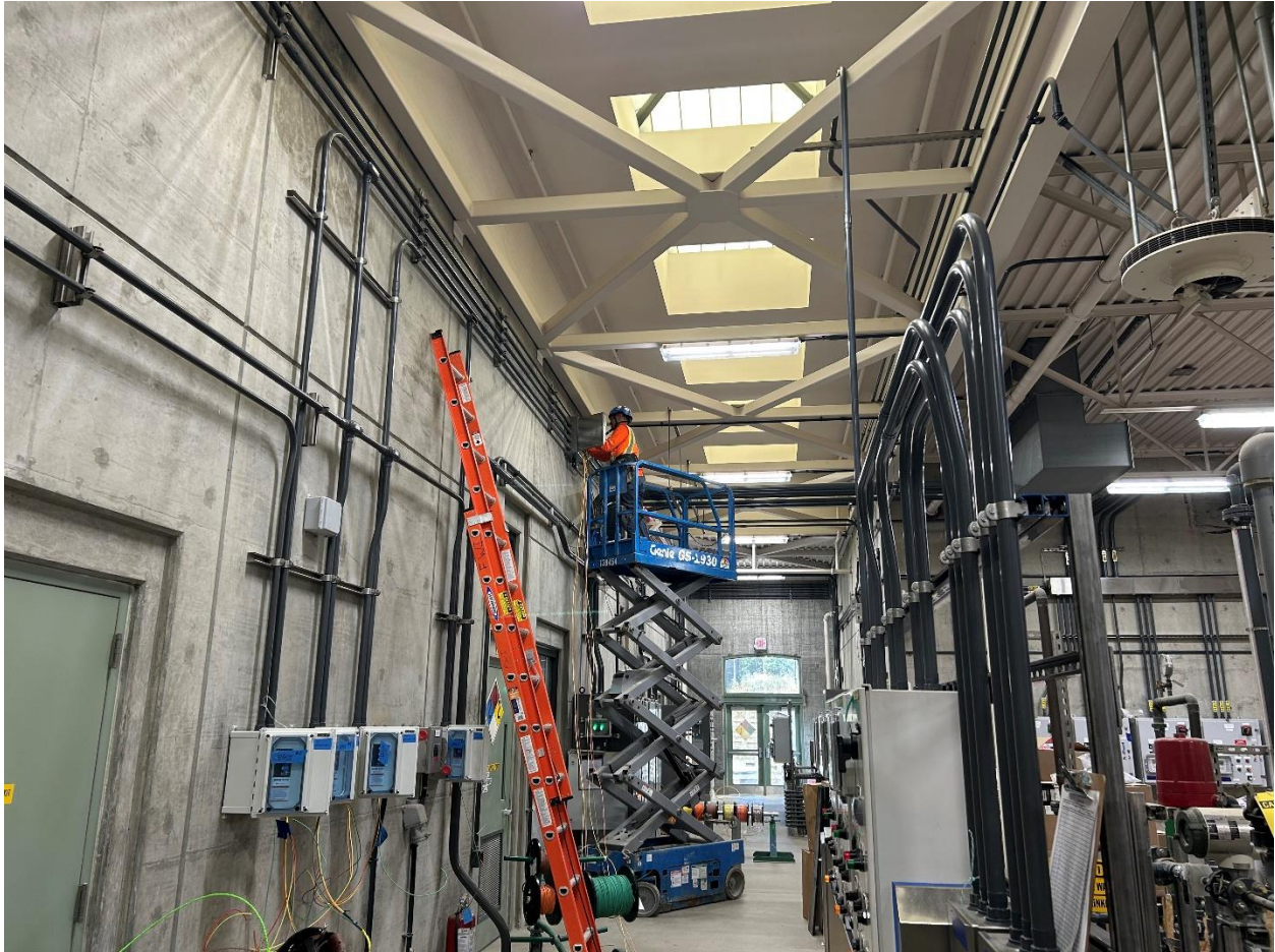
Photo 31 – Electrician on scissor lift in Chemical Building pulling electrical wires into conduits and pullboxes.
