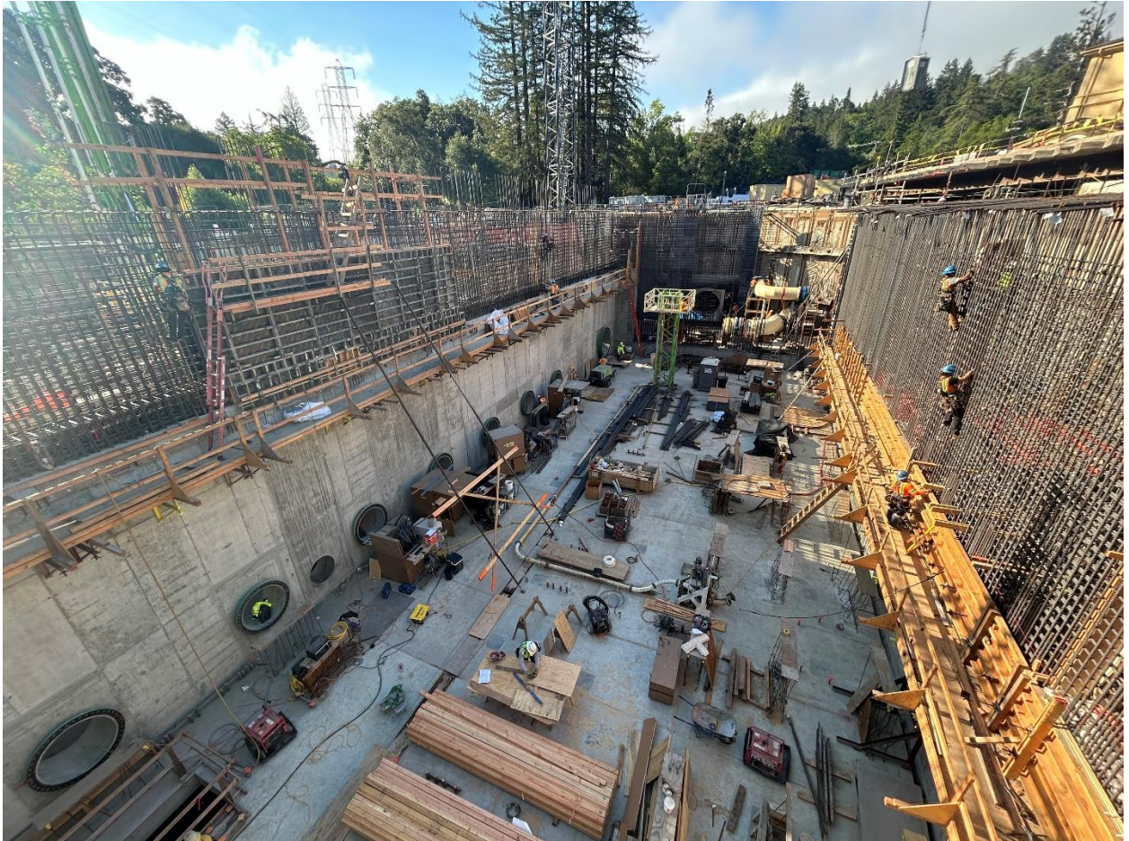
Photo 16 – View of the UV Room in the UV-CCB Facility starting to take shape. The effluent piping for the new UV disinfection vessels can be seen on the left wall. The valve vault can be seen in the far background of the UV Room.
