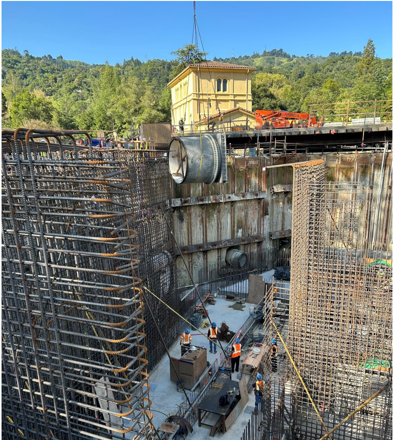
Photo 9 – The 108-inch piping and wall gate thimble being lowered into the UV-CCB with the aid of the 210-foot-tall tower crane.
