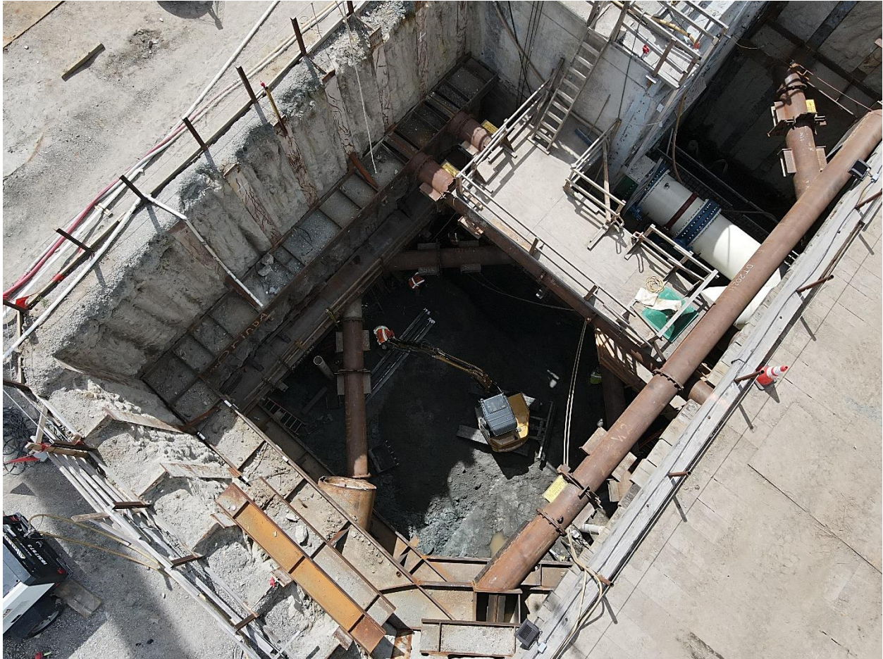
Photo 6 – Excavation 40-feet below ground surface in the Effluent 1 excavation pit in preparation for the 90-inch Effluent 2 tunnel. This pit is partially covered by the temporary construction bridge shown in the lower right-hand corner of the photo. The pit will have four piping tunnels and will serve as the key hydraulic connection point for connecting the existing filter plant to the new UV-CCB Facility.
