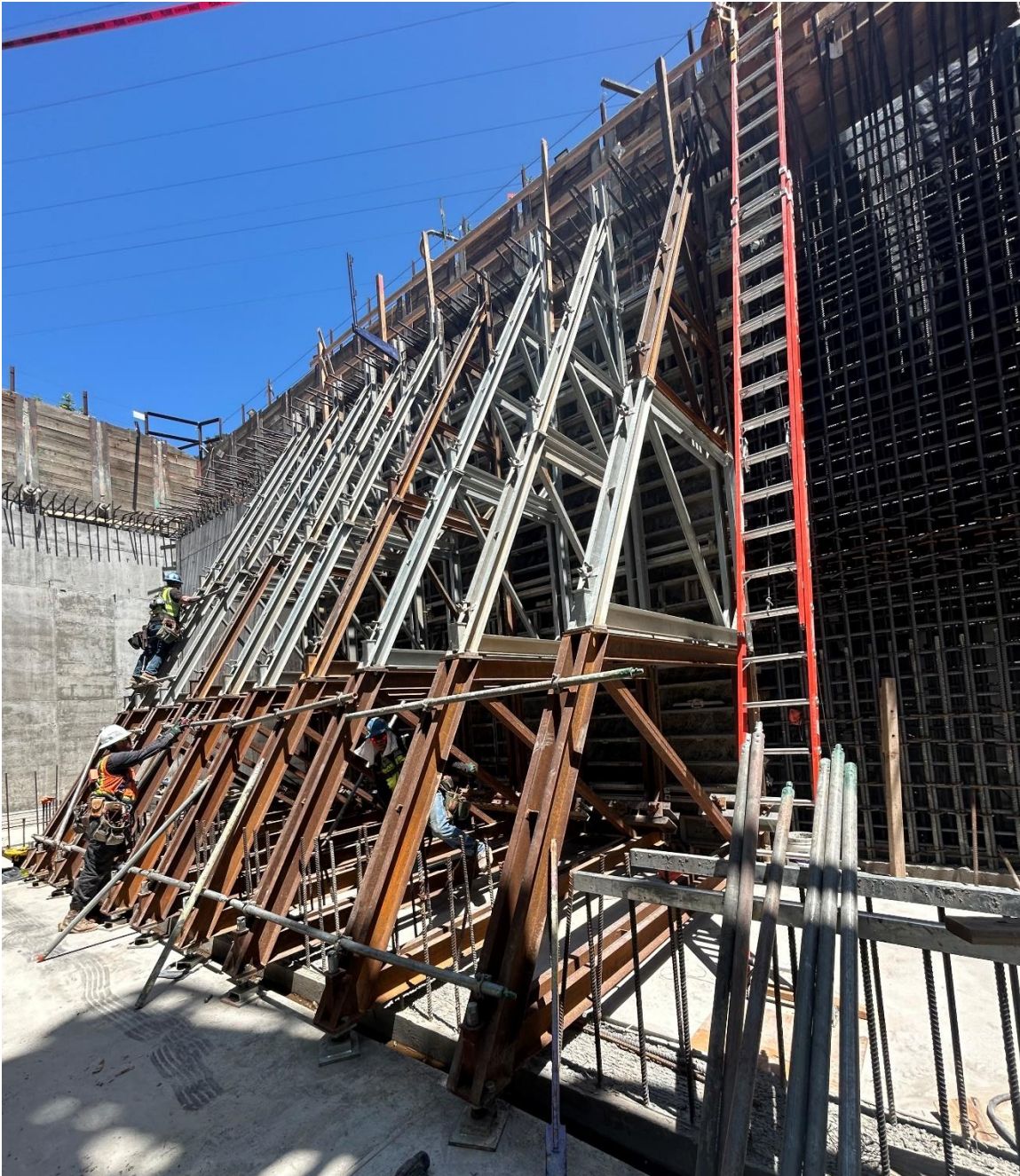
Photo 22 – Carpenters setting steel bracing for support the 25-feet tall concrete wall forms from buckling under the extreme pressure of the concrete placed into them.
