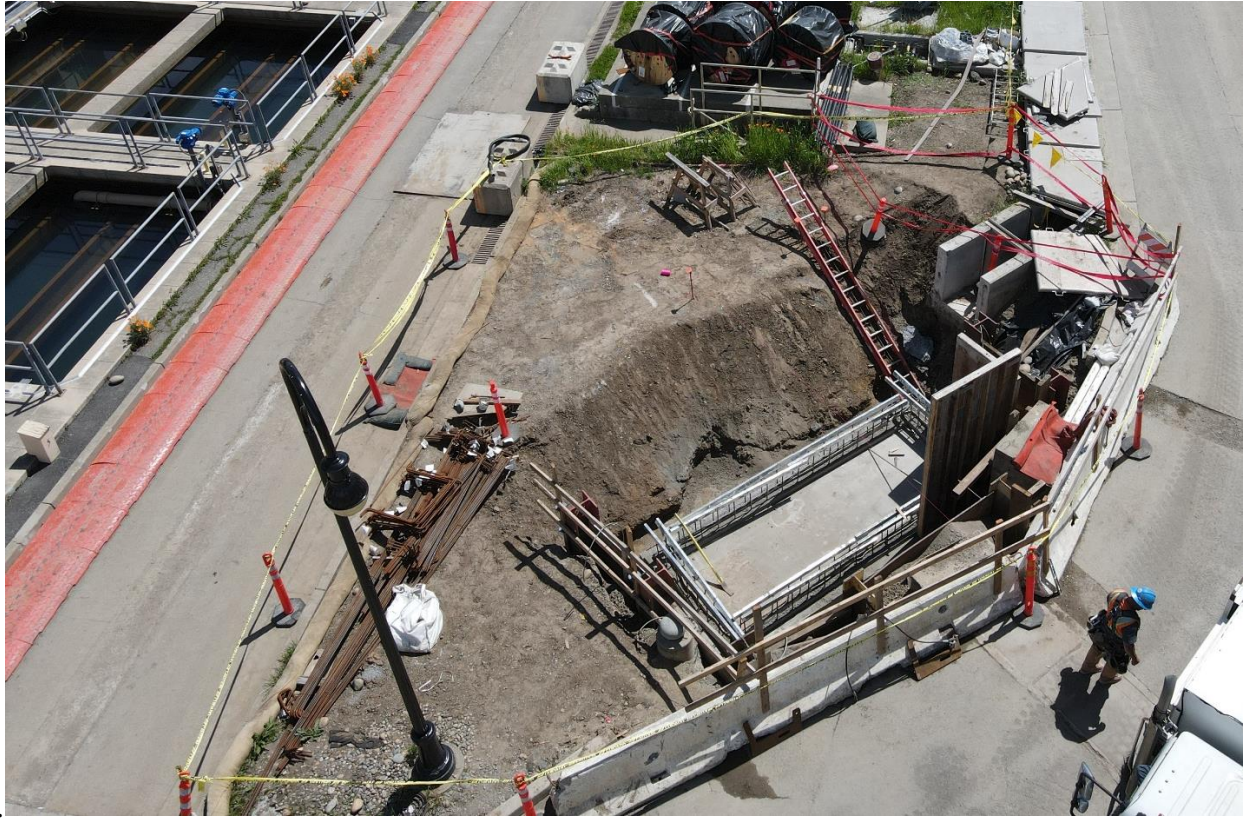
Photo 27 – Aerial view of excavation and concrete foundation for the new chemical sump which safely contain chemical spills.
