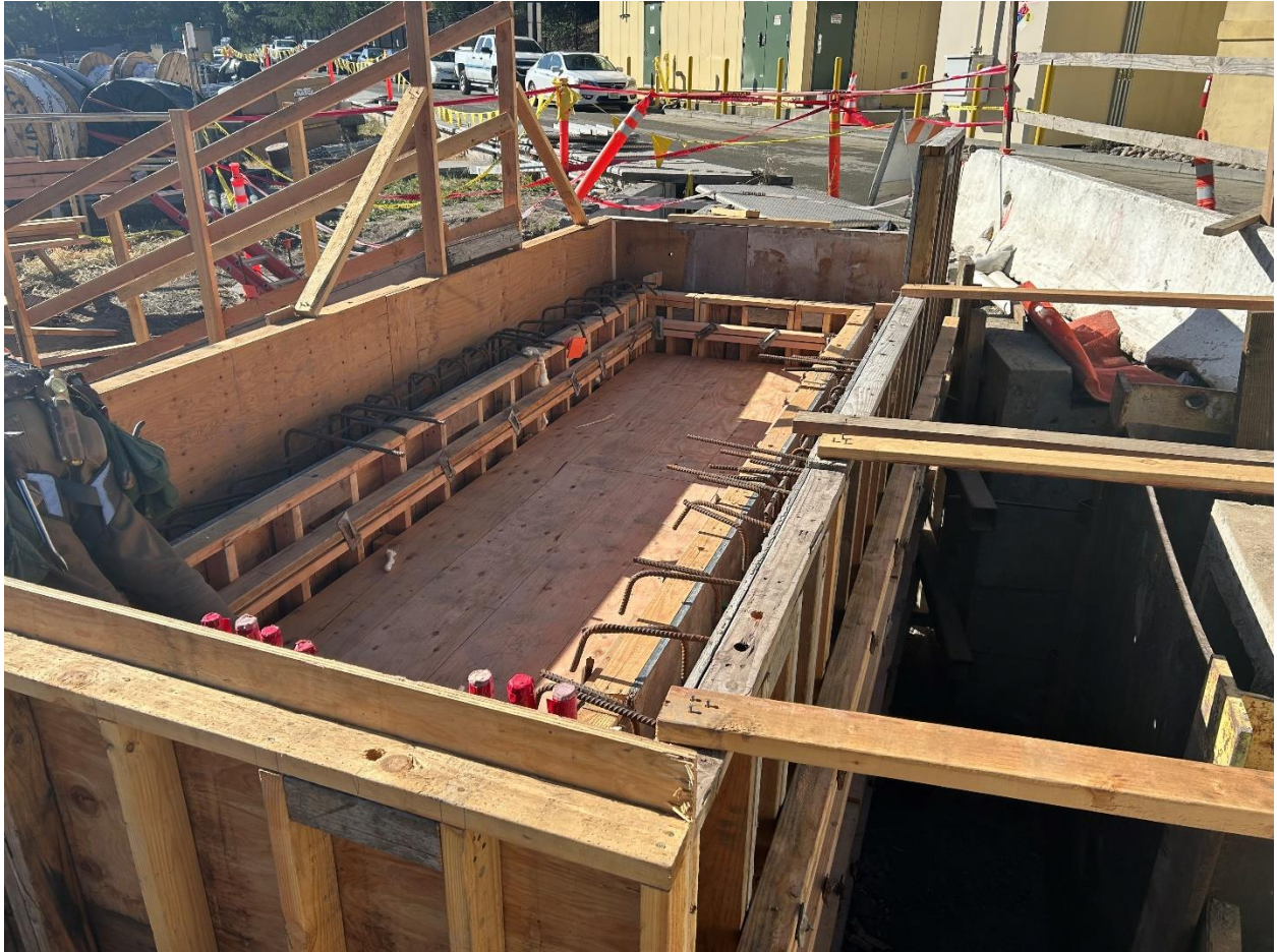
Photo 28 – Closeup view of concrete formwork for the new chemical sump 2 which will contain future chemical spills that arise from leaking pipes in the adjacent chemical trenches.
