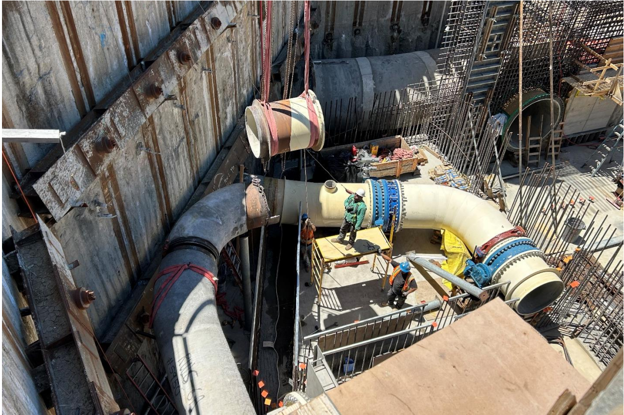
Photo 13 – Pipefitter positioning a section of the 36-inch wasteway piping within the valve vault of the UV-CCB Facility with the aid of the tower crane. The photo shows the complexity of the piping and valving in the valve vault.
