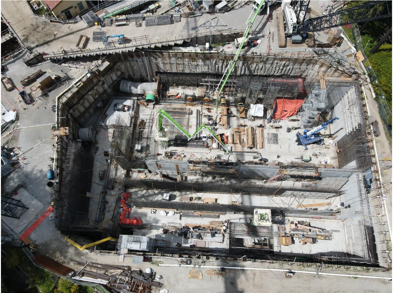
Photo 15 – Aerial view of the UV-CCB excavation pit with the underground structures starting to take shape. The foundation for structures are 65-feet below the ground surface.
