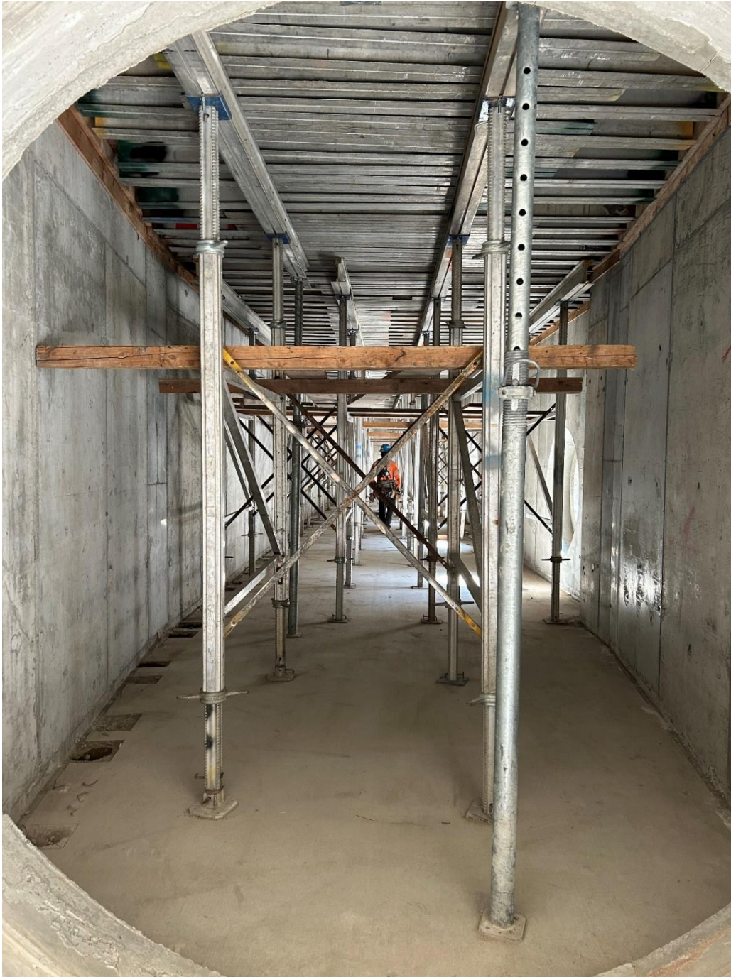
Photo 24 – Portal from the 108-inch UV-CCB influent piping into the UV Influent Weir Structure. The aluminum shoring and decking shown in the photo supports the weight of the concrete roof until it attains proper strength after curing. The UV Influent Weir Structure will provide even flow to each of the UV vessels located in the UV Room to the right of the photo.
