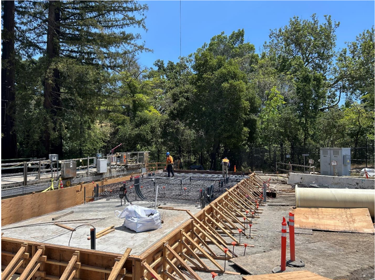
Photo 4 – Ironworkers installing rebar for the future Los Altos Power Building foundation which is located on top of the former Los Altos Pumping Plant No. 1 (LAPP1). All remnants of the intricate underground piping installed in the former LAPP1 are backfilled below the foundation in the photo.
