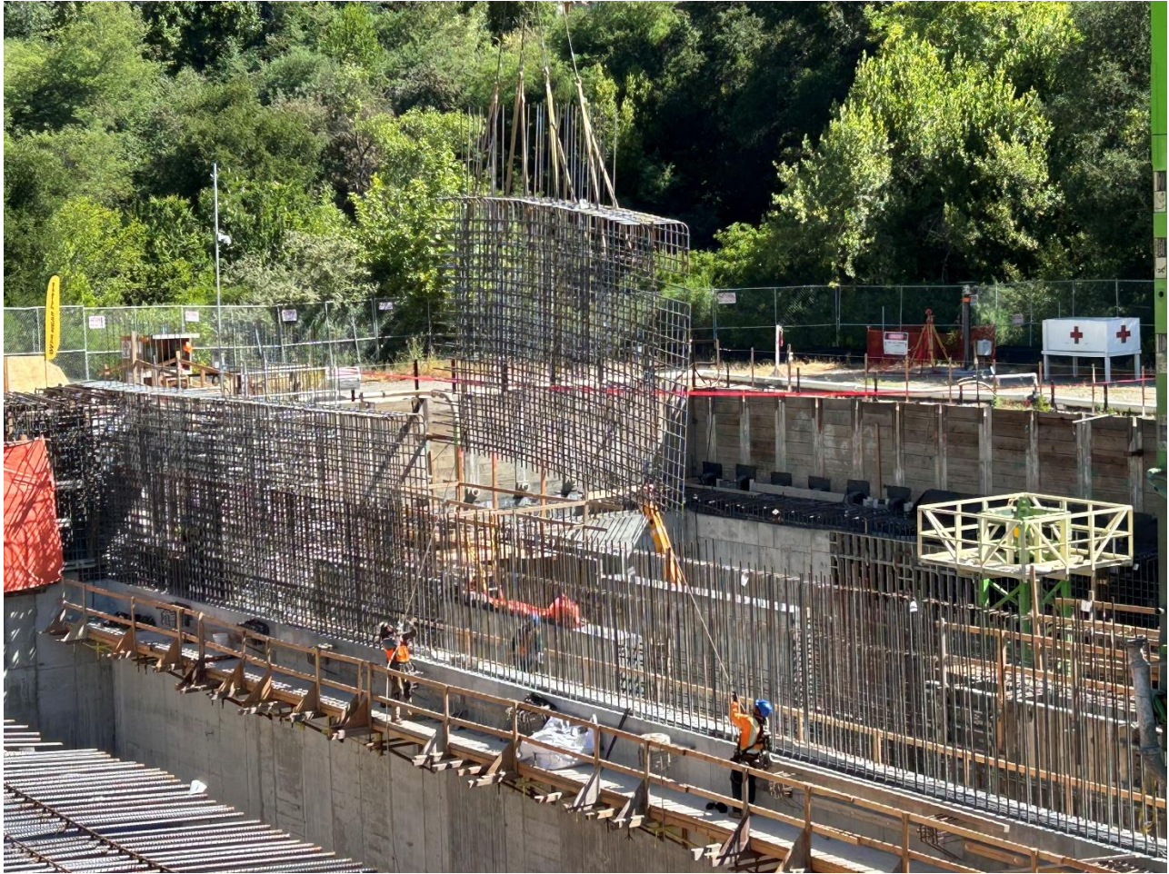
Photo 17 – Ironworkers lowering a prefabricated rebar curtain into position at the divider wall between the Chlorine Contact Basin and the UV Room in the UV-CCB Facility.
