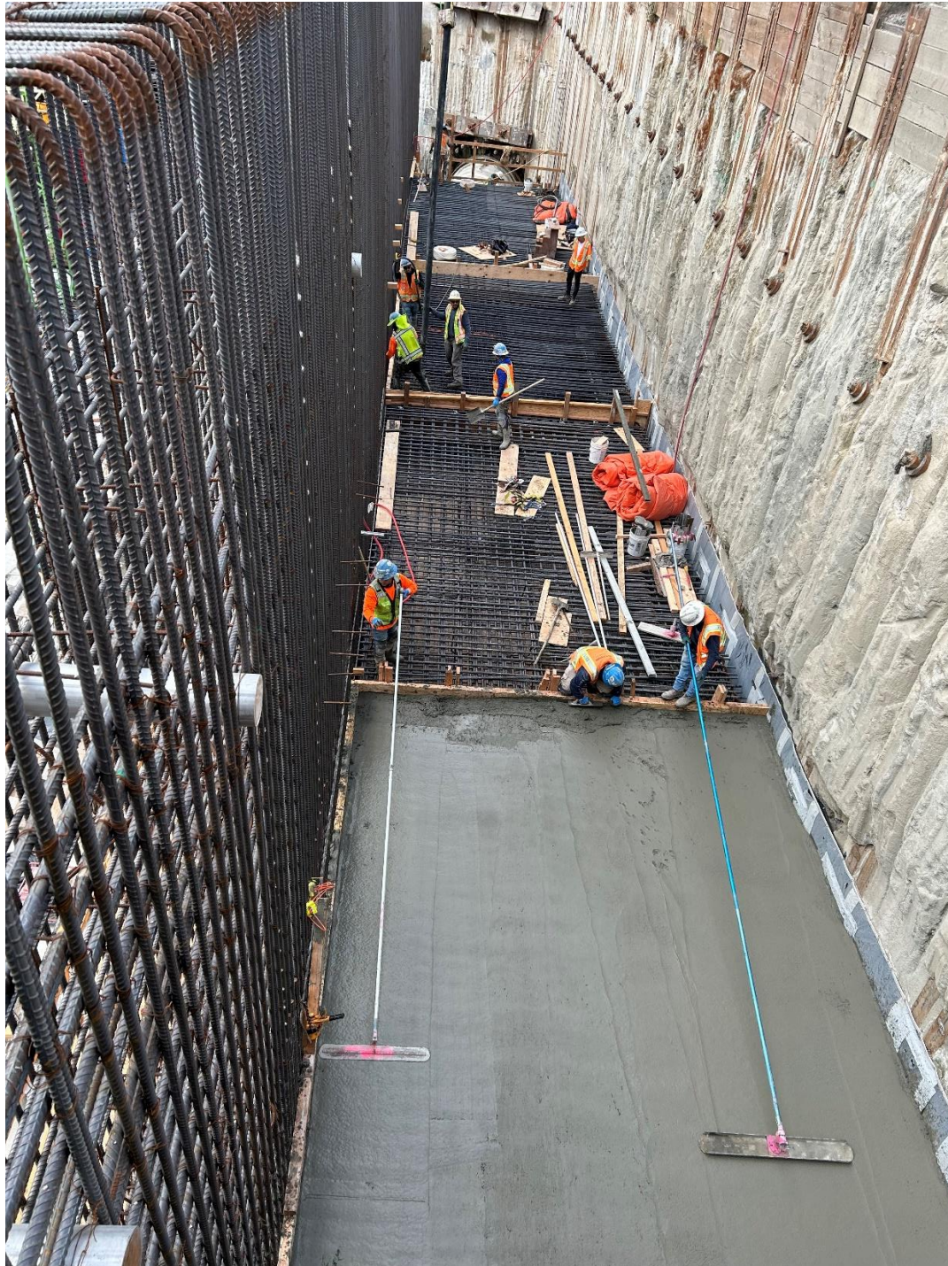
Photo 25 – Finishers placing concrete for the UV Influent Weir Structure roof deck. The rebar for the exterior wall of the UV Room is on the left side of the photo and the excavation support system is shown on the right side of the photo.
