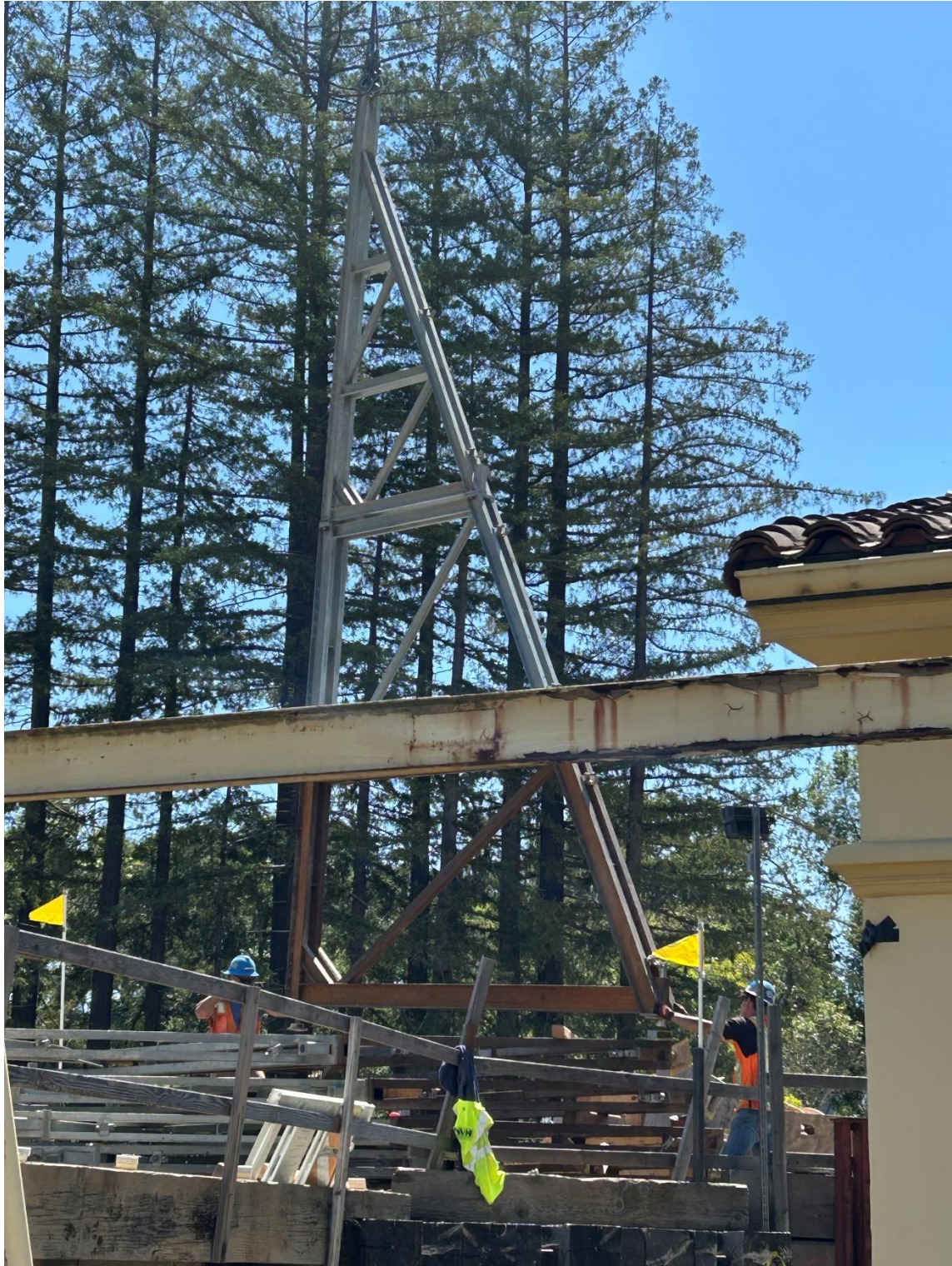
Photo 21 – Carpenters setting down a massive steel bracing with the aid of the tower crane. These bracing segments are engineered to support the 25-foot tall concrete wall forms.
