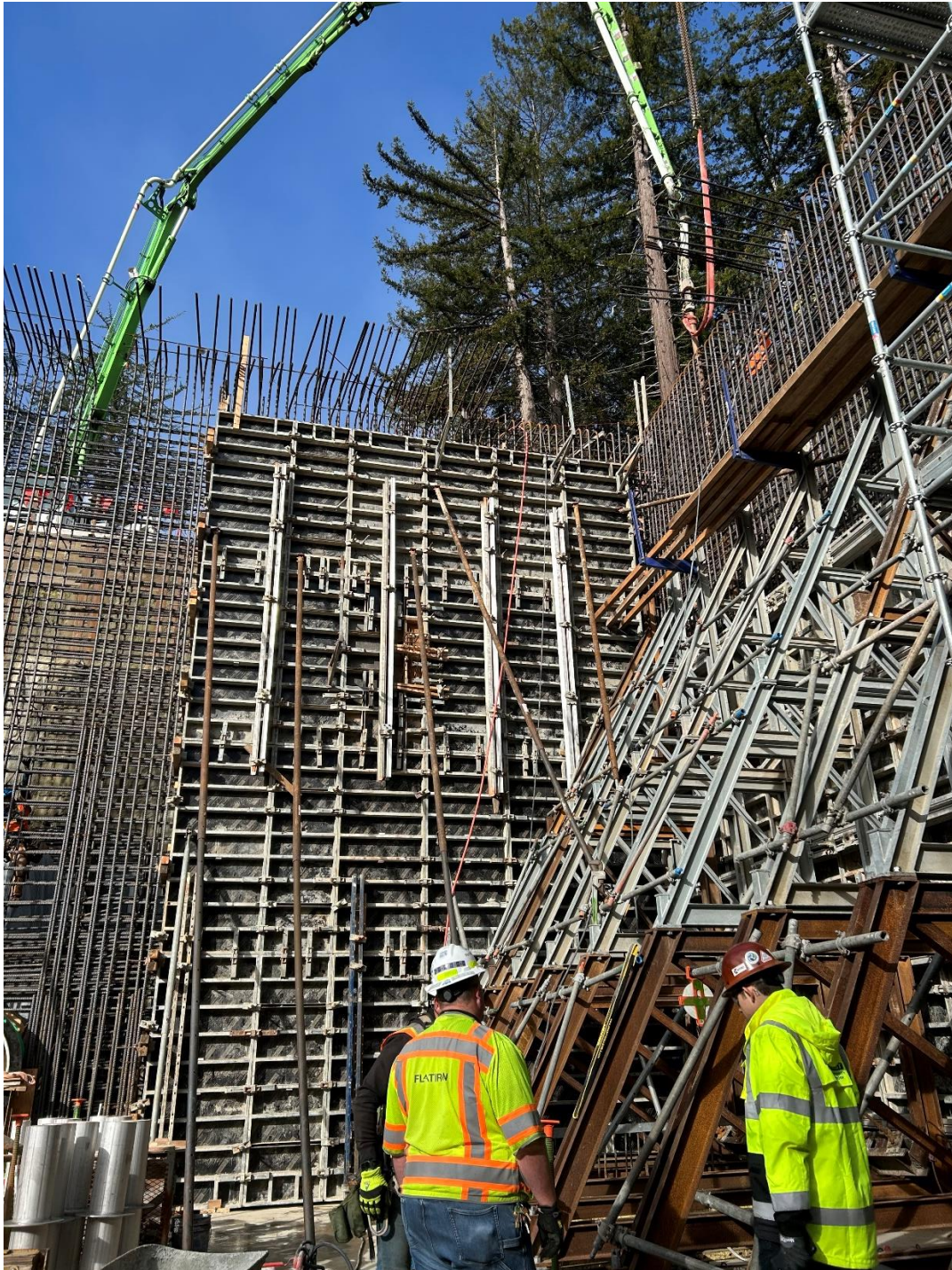
Photo 23 – Placing concrete into the first exterior UV Room wall. The green concrete pumping truck with its articulating boom can be seen at the top of the photo placing concrete into the 25-foot tall concrete wall forms.
