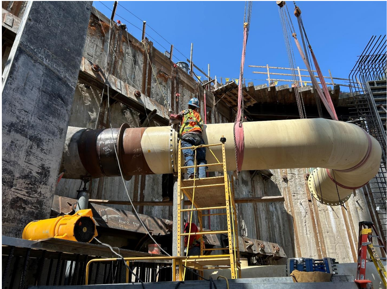
Photo 12 – Pipefitter positioning the 36-inch wasteway piping within the valve vault of the UV-CCB Facility with the aid of the tower crane.
