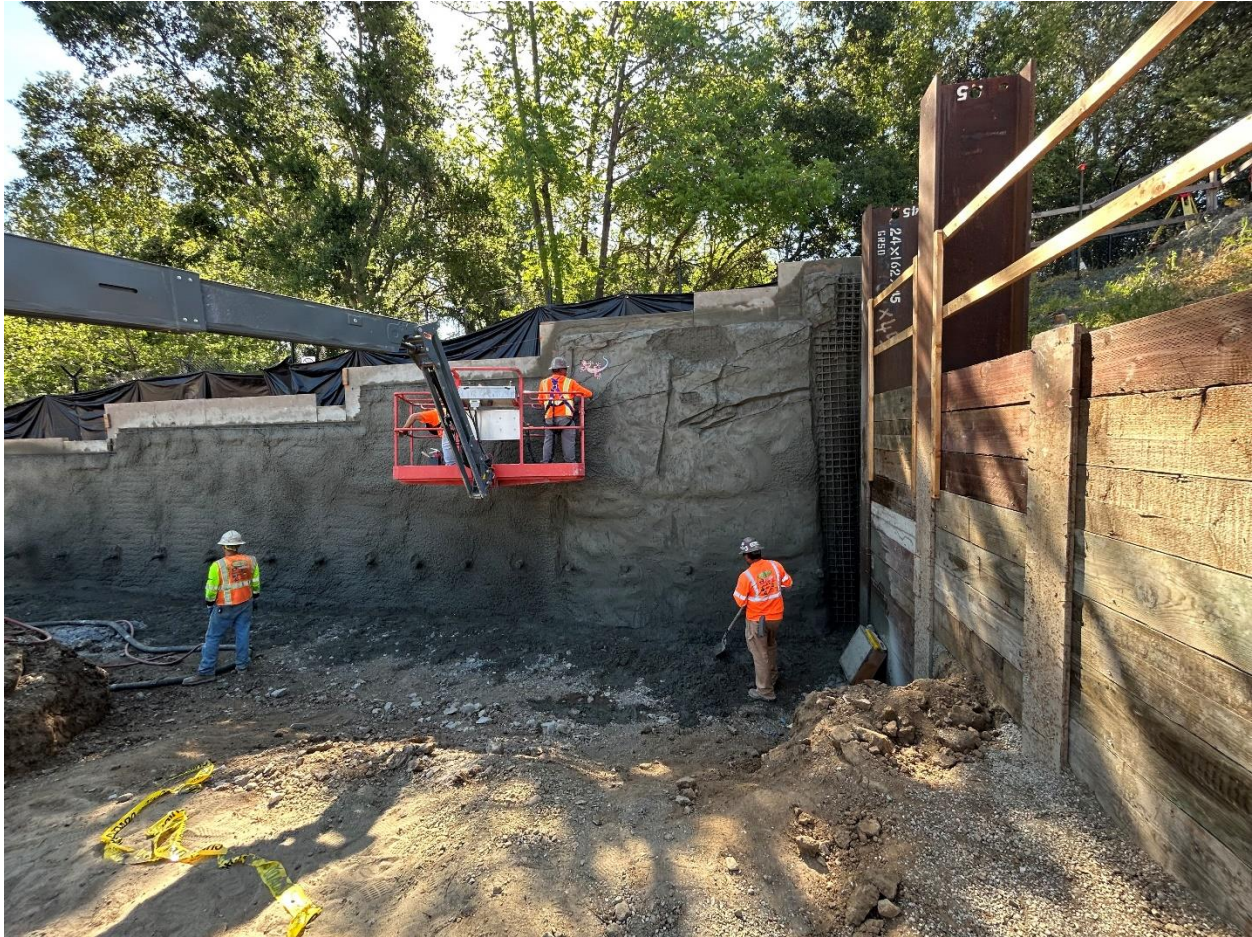
Photo 1 – Masons applying architectural finish to the shotcrete retaining wall.
