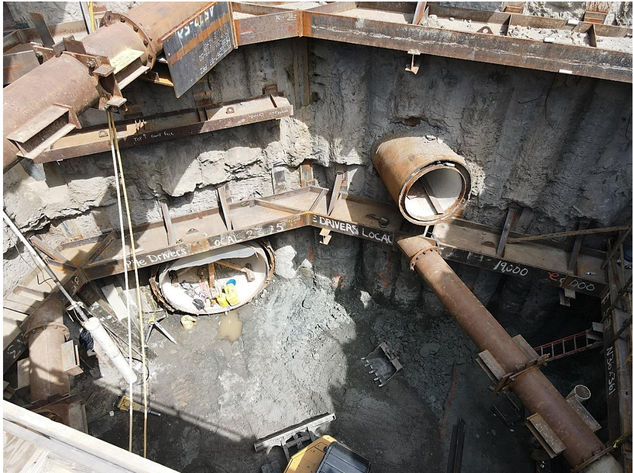
Photo 7 – Closeup of Effluent 1 excavation pit showing the complex welded steel pipe and beam shoring system. The lower left tunnel has the 108-inch UV-CCB influent pipe and the upper right tunnel has the 48-inch effluent pipe for Los Altos Pumping Plant No. 2.
