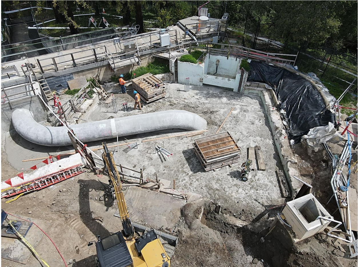
Photo 3 – Aerial view of former Los Altos Pumping Plant No. 1 backfilled with slurry. Emergency 48-inch raw water bypass piping is shown aboveground in this photo.
