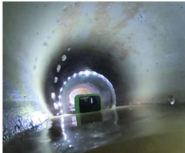
Camera in sewer during inspection
