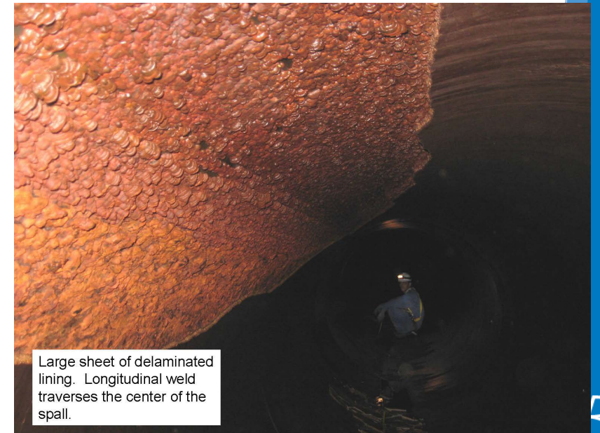
Internal Corrosion of Steel Pipe at CML Failure
