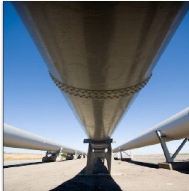
Aboveground Section of Mokelumne Aqueduct
