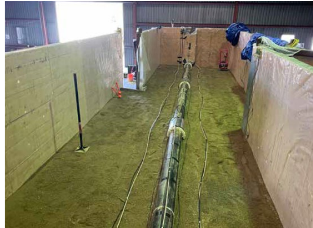
Split Basin before Backfill
