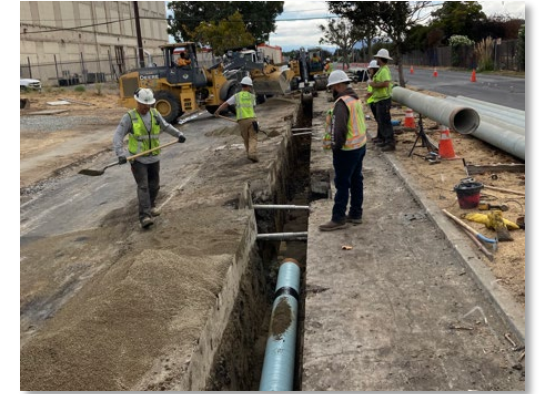
Steel Pipe Installation
