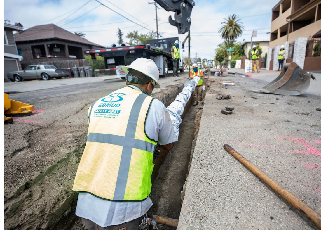
Ductile Iron Pipe Installation
