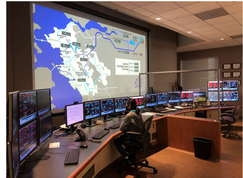
Oakland Control Center, Administration Building
