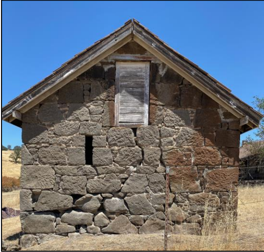
Wildermuth House Granary before repointing
