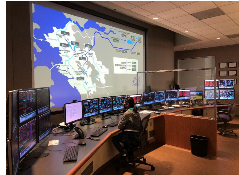
Oakland Control Center, Administration Building
