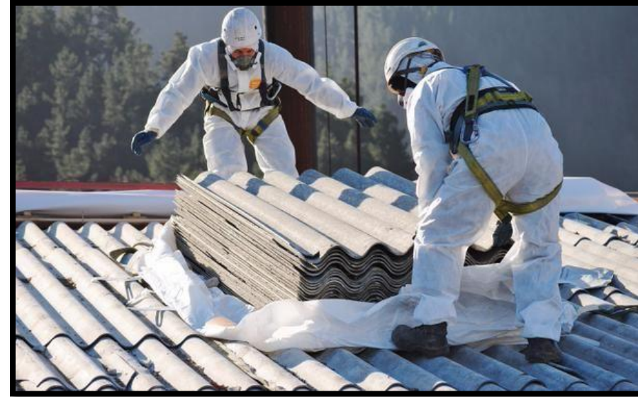
Workers removing roof tiles with hazardous materials
