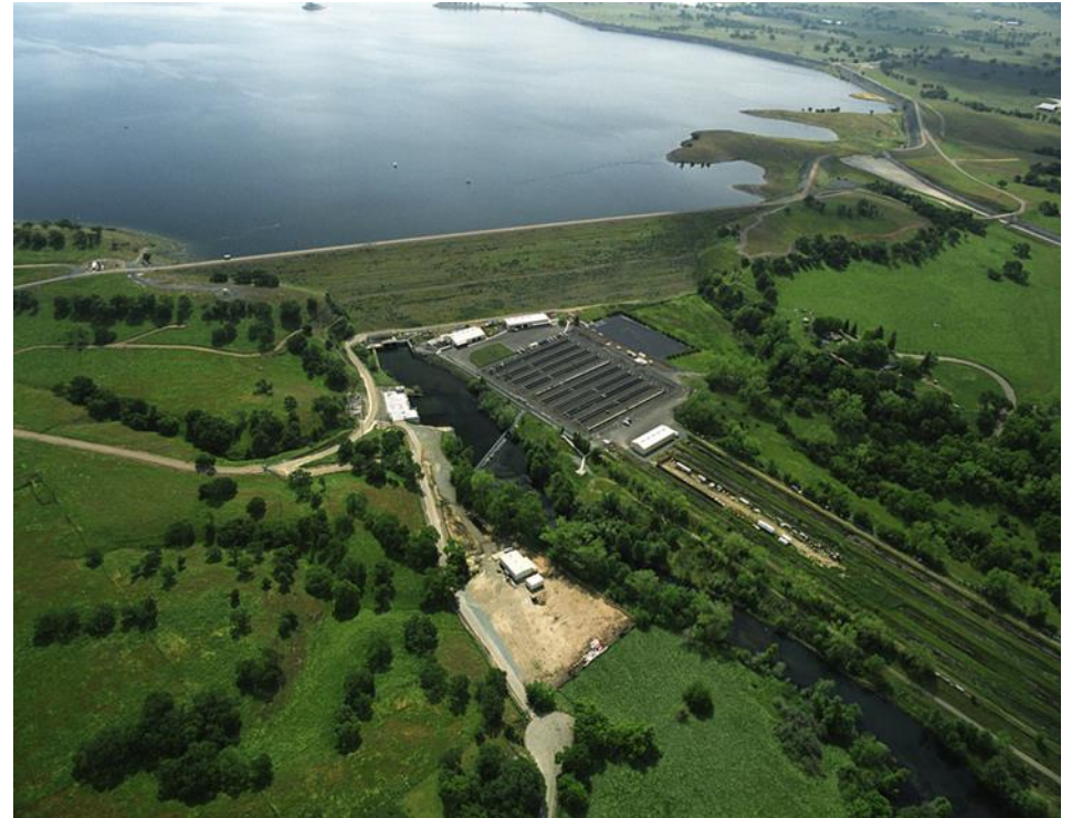
Aerial Photo of Camanche Dam and Hatchery
