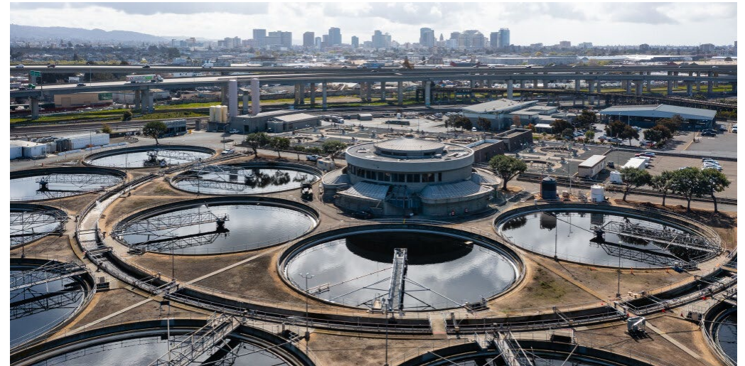
Overlooking the Main Wastewater Treatment Plant, looking southeast towards Downtown Oakland
