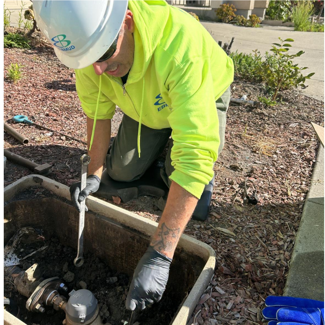
District staff replacing a meter
