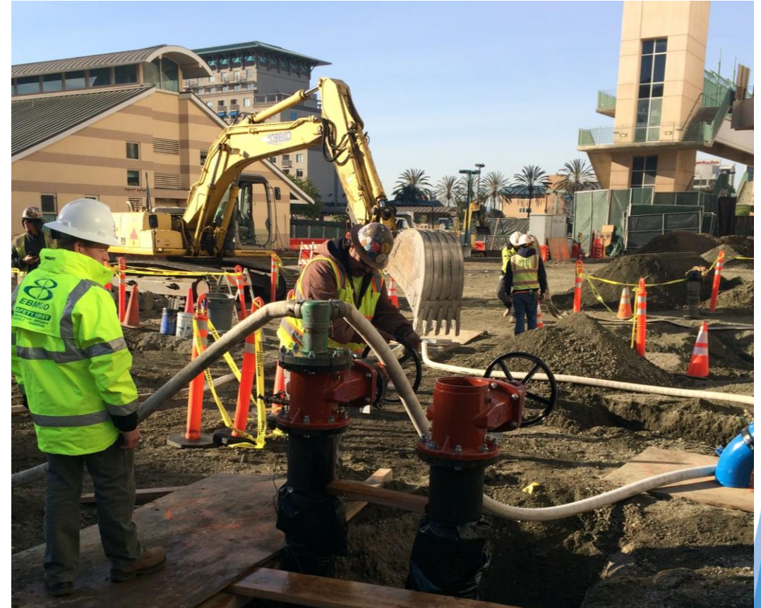
District staff inspecting new construction
