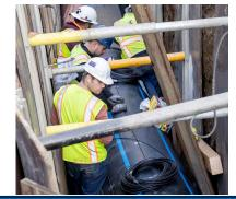
Fiber Optic Cable Installation on Summit Pipeline in Berkeley
