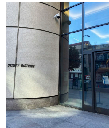
Security Camera Upgrades (AB and AMC)
