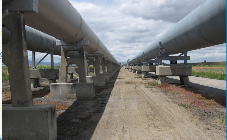
Mokelumne Aqueducts Nos. 1, 2, & 3 in the Delta
