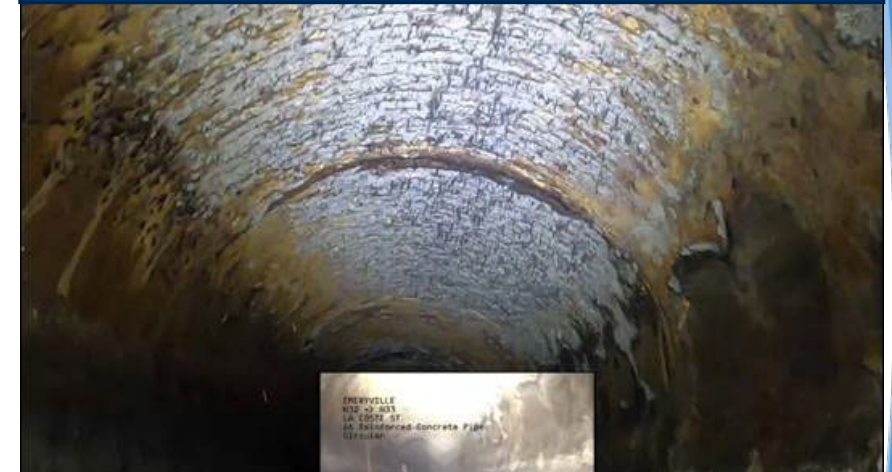
Corroded Maintenance Hole
