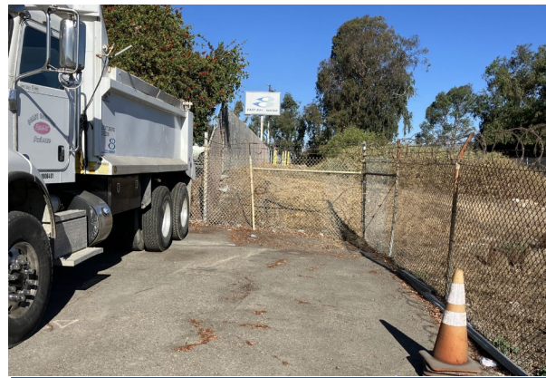
Fencing and Security Improvements (Oakport)
