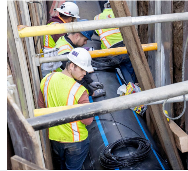
Fiber Optic Cable Installation on Summit Pipeline in Berkeley
