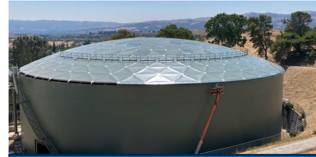
Castenada Reservoir No. 1
