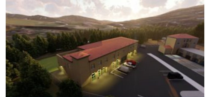
New Consolidated Maintenance and UV Building
