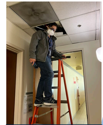
AB Ceiling Inspections for Future Fire Wall Repairs
