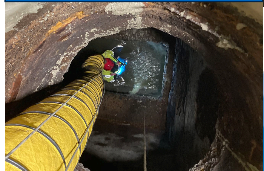
Corroded Maintenance Hole
