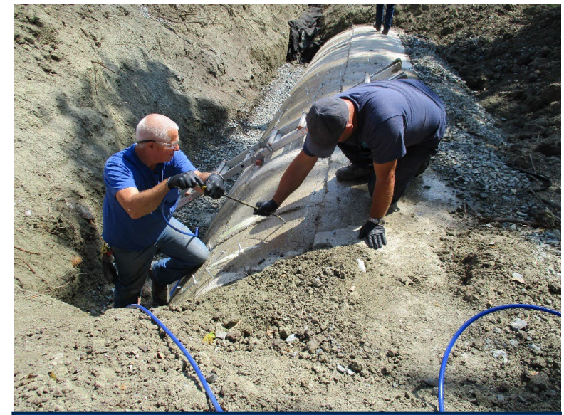
District Forces Repairing Leak on LAF 1 Pipeline
