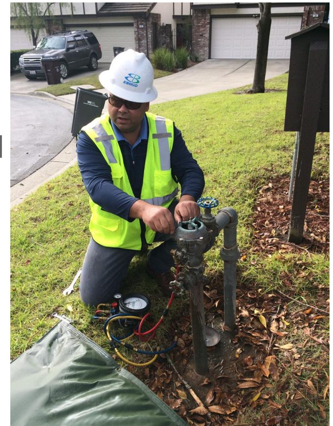
District staff working on a backflow prevention assembly
