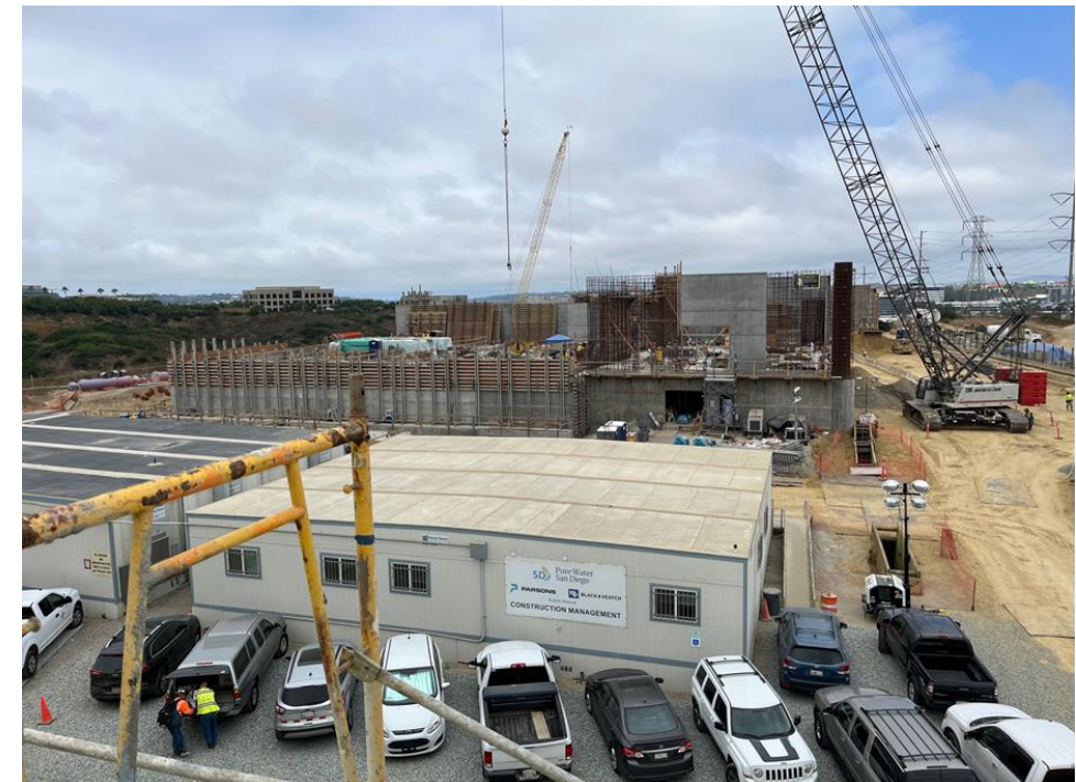
Pure Water San Diego construction site Photo courtesy of F. Wedington
