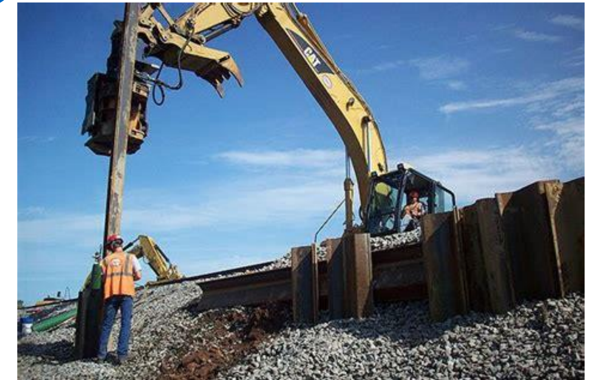
I-Beam Installation
