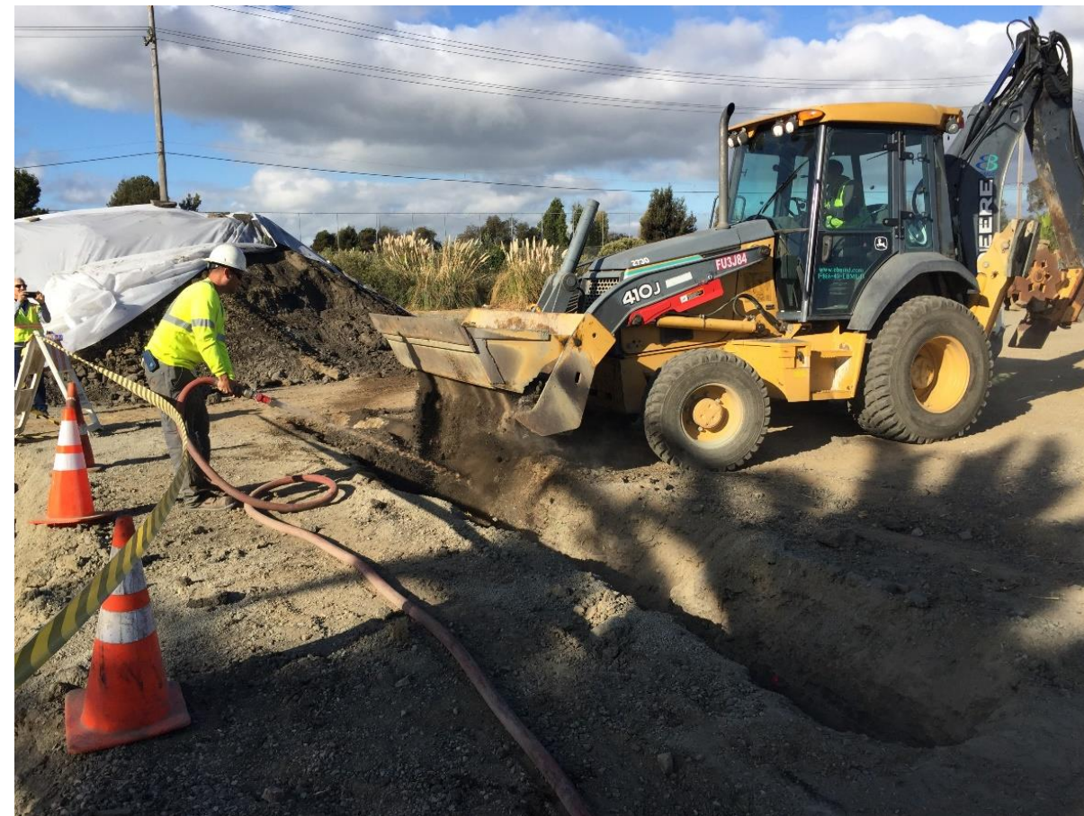
Amending Native Soil for Reuse in Trench
