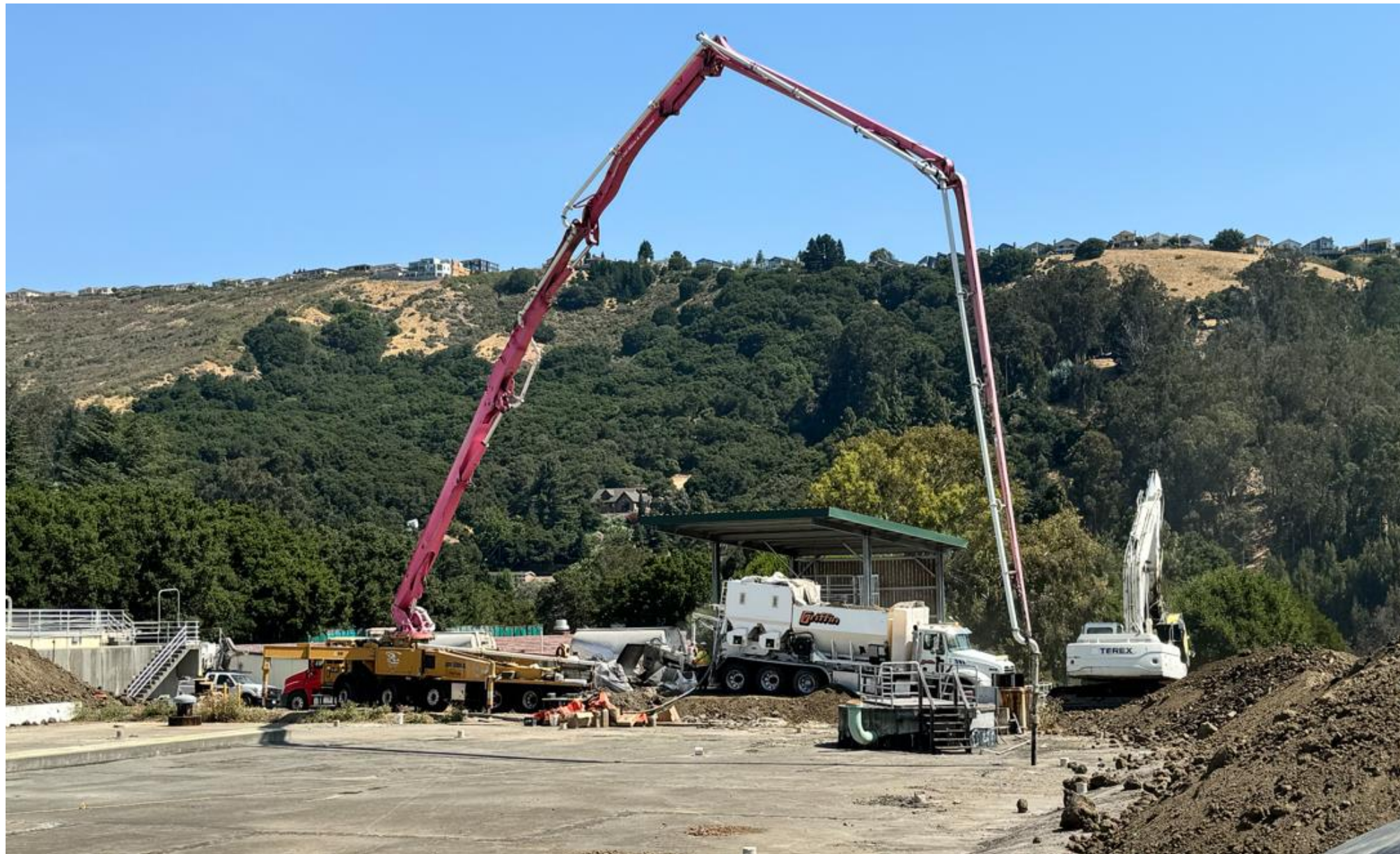
Pumping native slurry in chlorine contact basin
