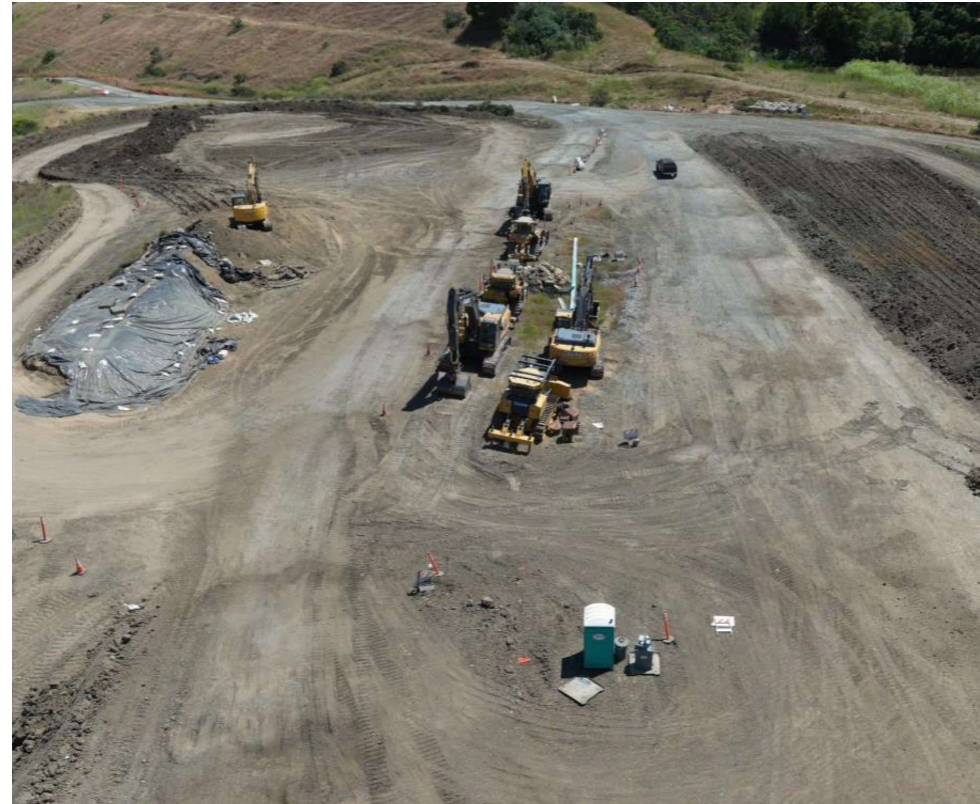
Briones Trench Soil Stockpile
