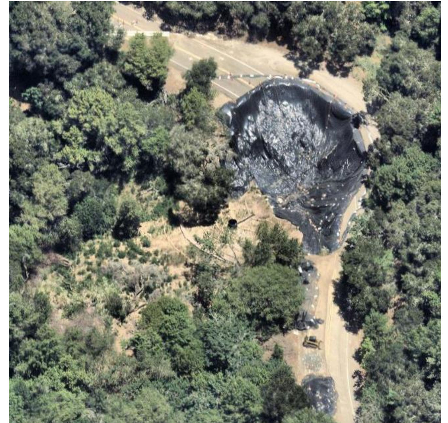
Redwood Road near Miller Road
