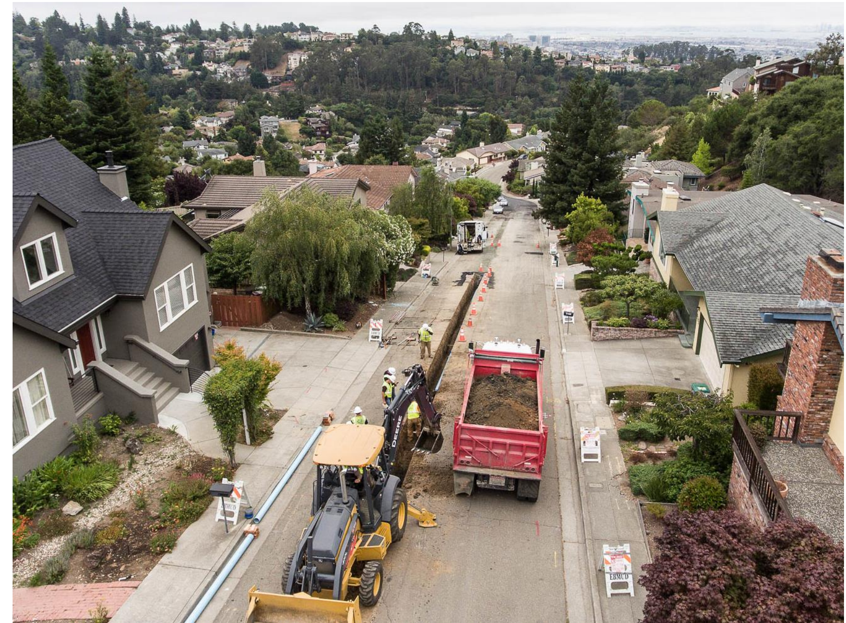
Typical Pipeline Construction
