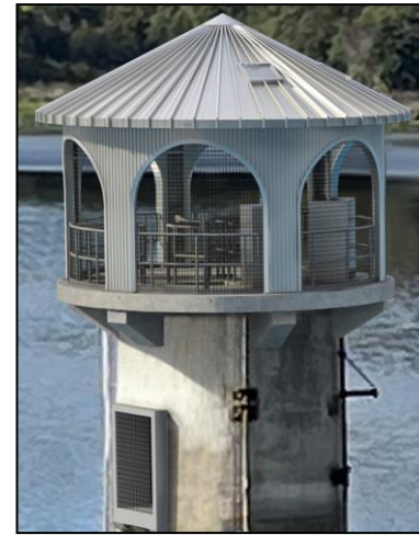
Metal Operating House
