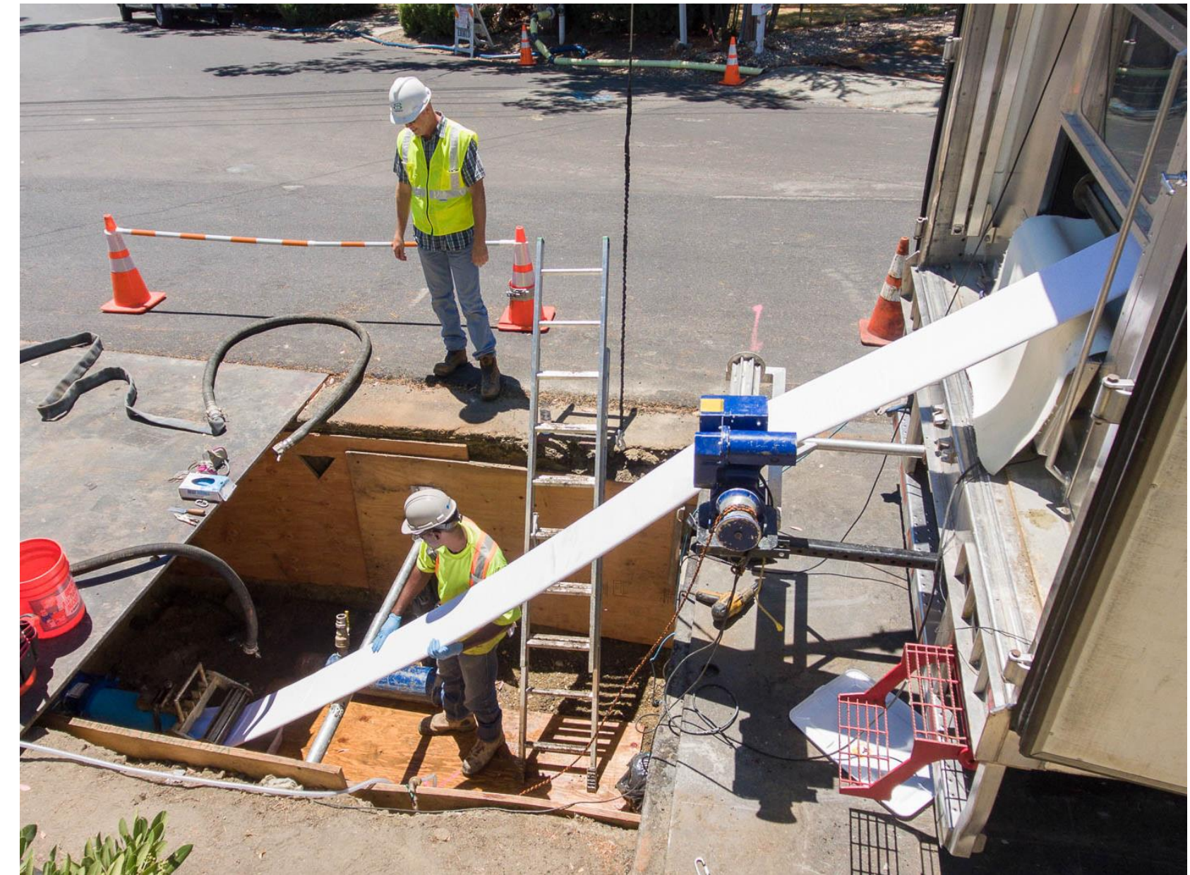
Installation of CIPP Liner
