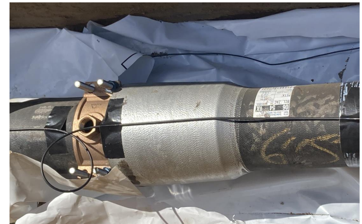
Fiber optic installation on ERDIP (Le Roy Cluster)
