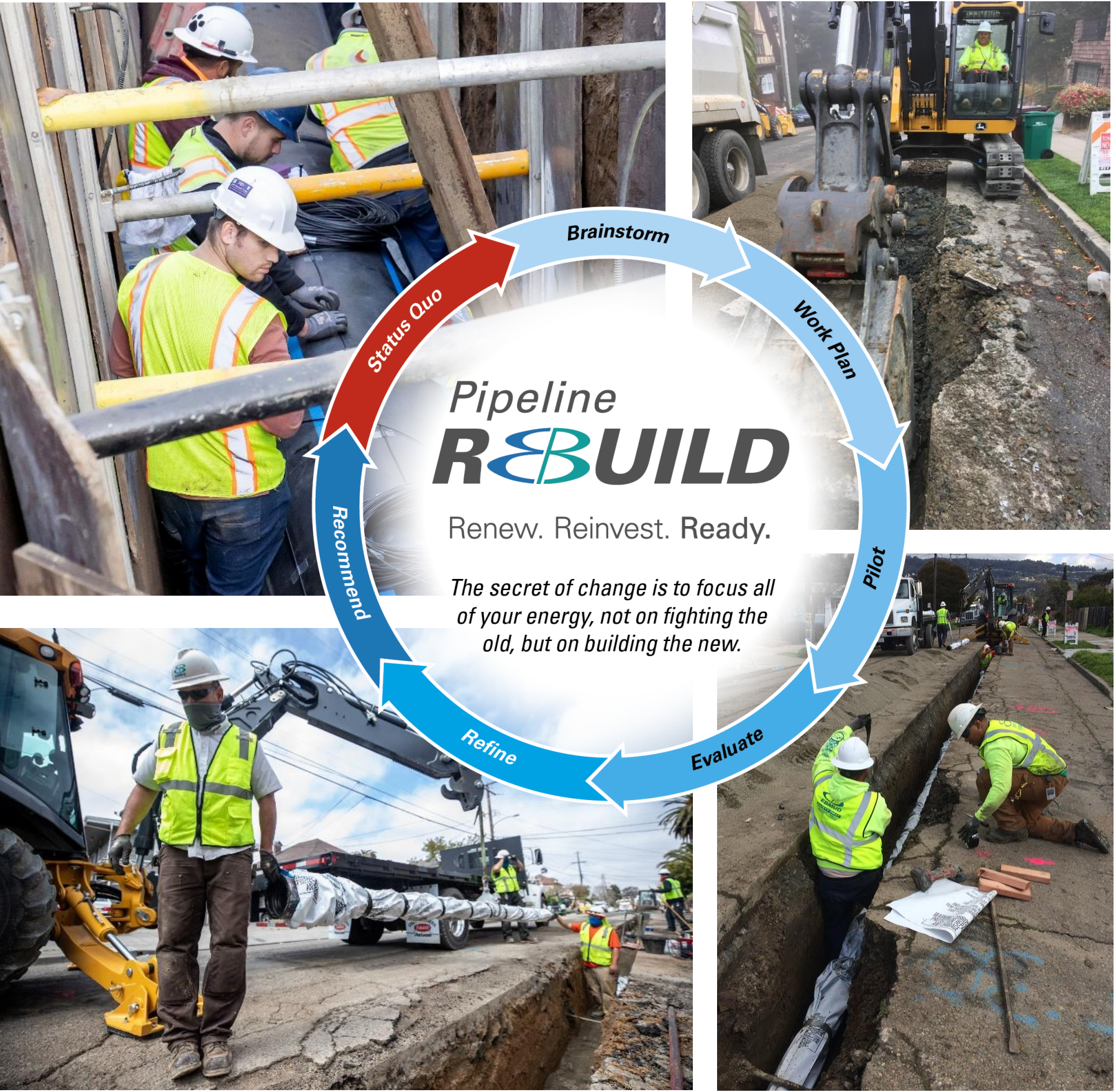
District Pipeline Construction
