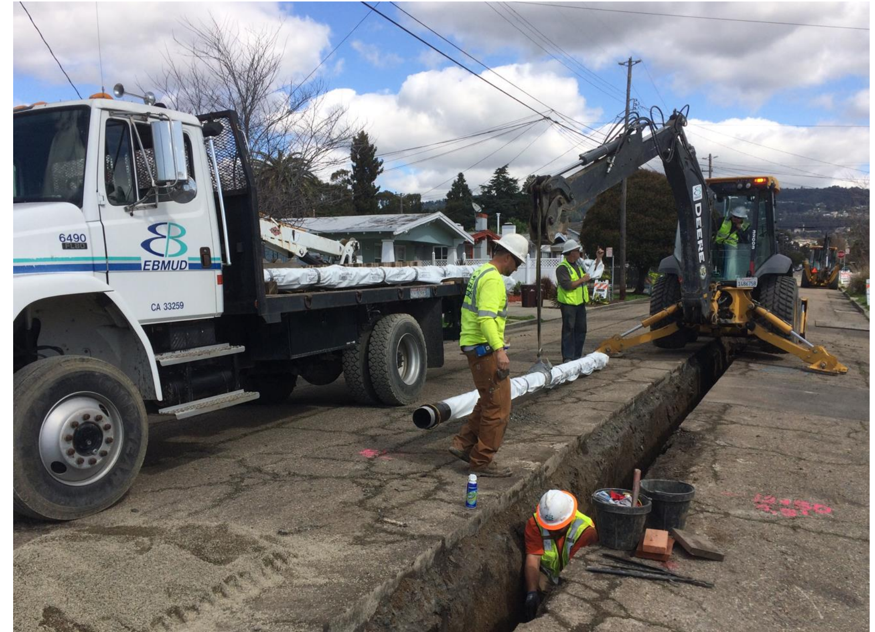
Pipeline Construction crews installing ductile iron pipe
