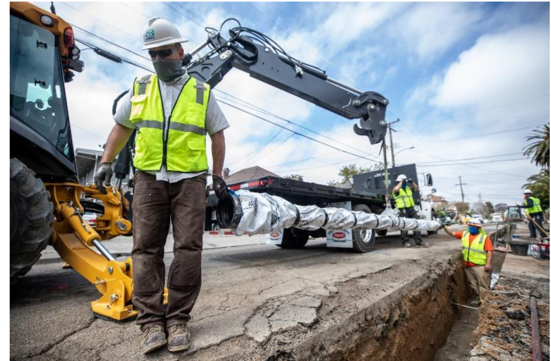
Ductile Iron Pipe Installation
