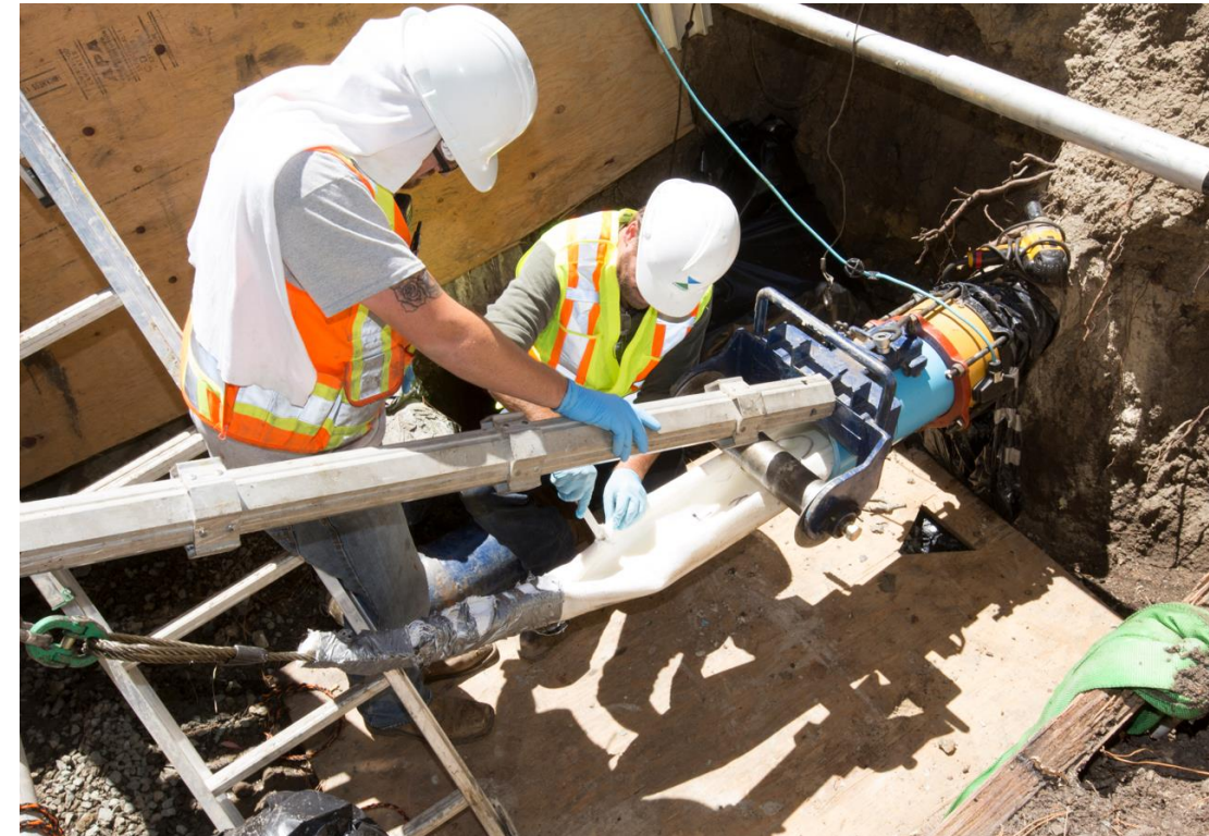
CIPP liner installation
