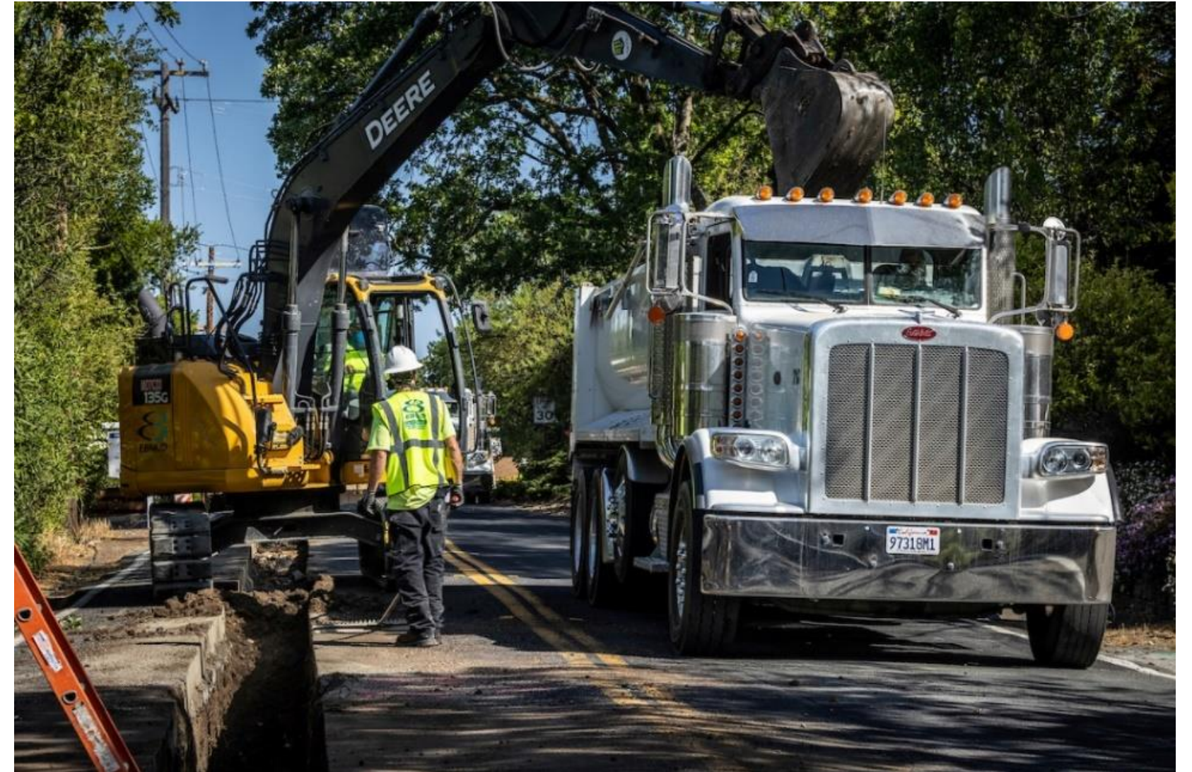
District Pipeline Construction
