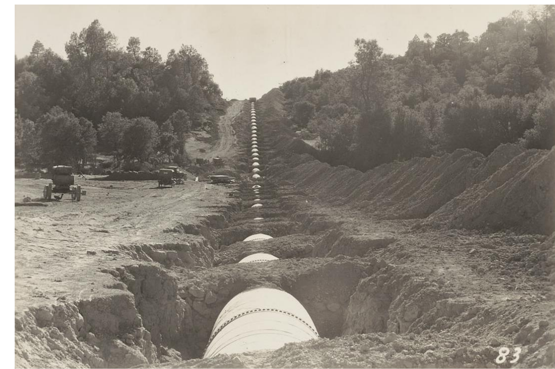
Mokelumne Aqueduct Construction (circa 1929)
