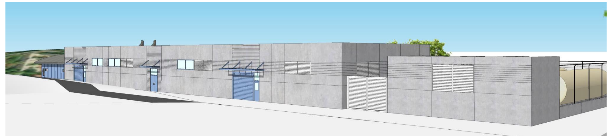
Ozone Generation Building
