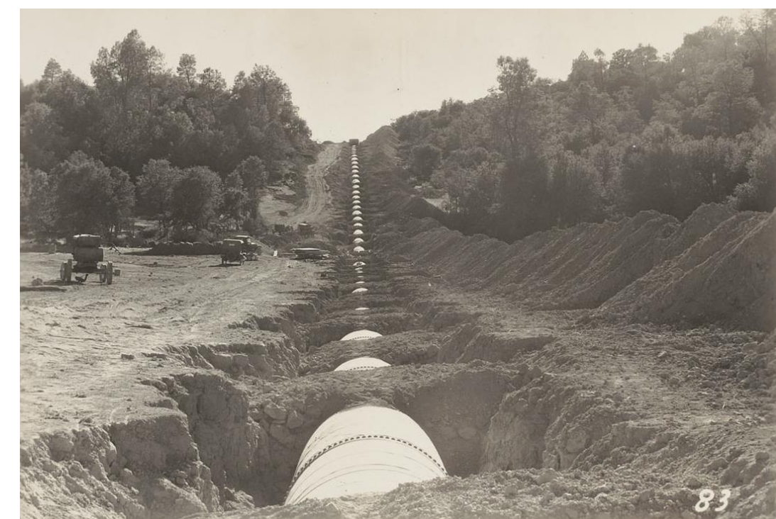
Mokelumne Aqueduct Construction (circa 1929)
