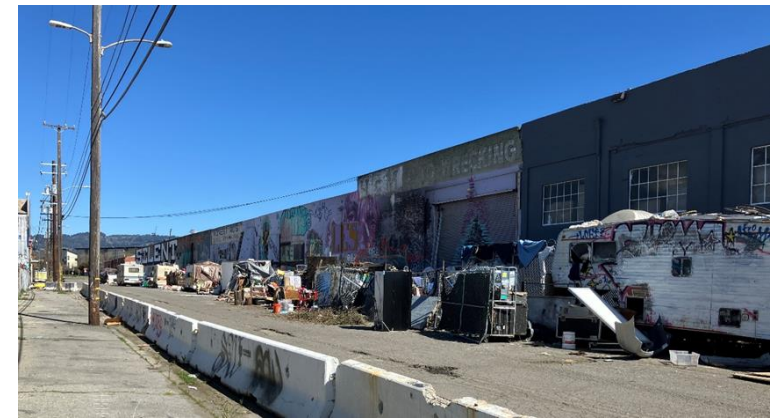
Existing Conditions on Willow Street
