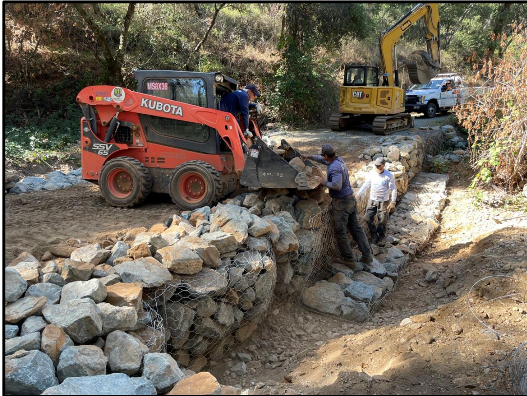
Middle Bar, Pardee Watershed Road Repair October 2023
