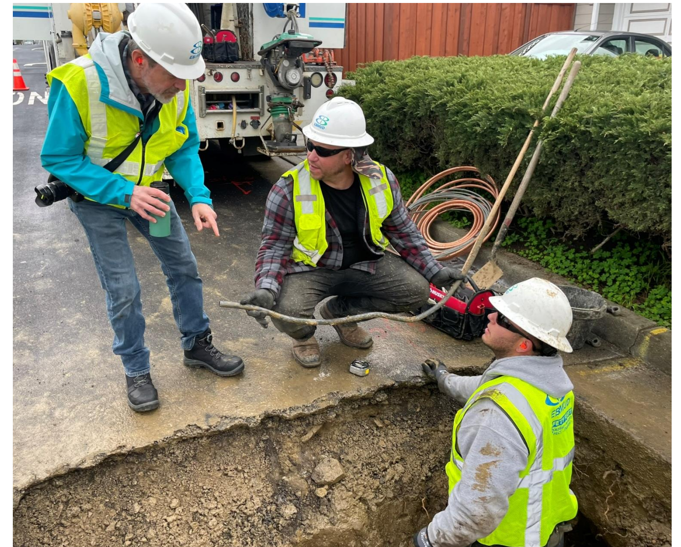
District staff replacing a service line
