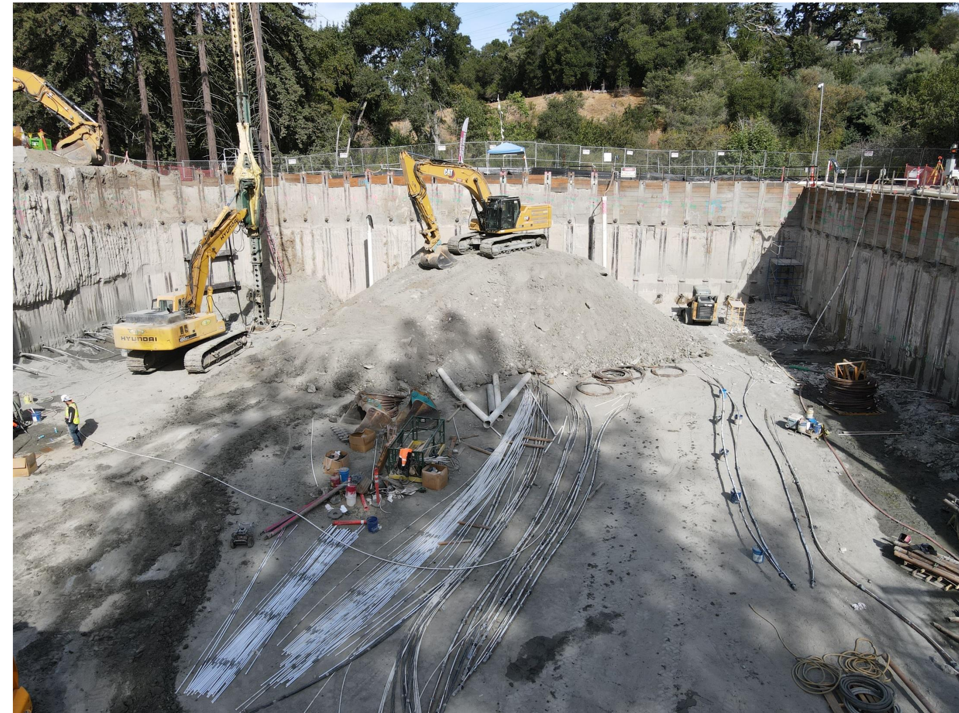
Excavation site at Orinda WTP
