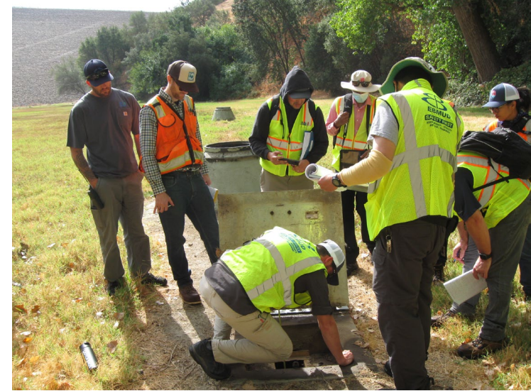
Annual FERC Inspection at Camanche Dam in 2023
