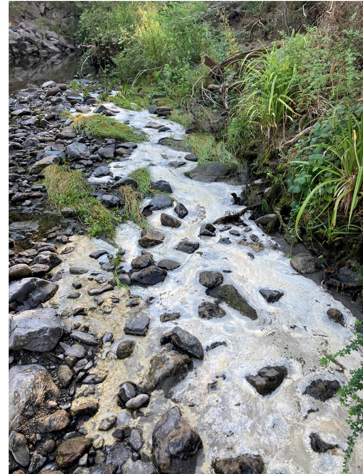
Grout release into San Pablo Creek
