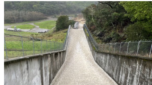
USL Reservoir Spillway
