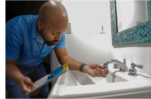
Installing a faucet aerator
