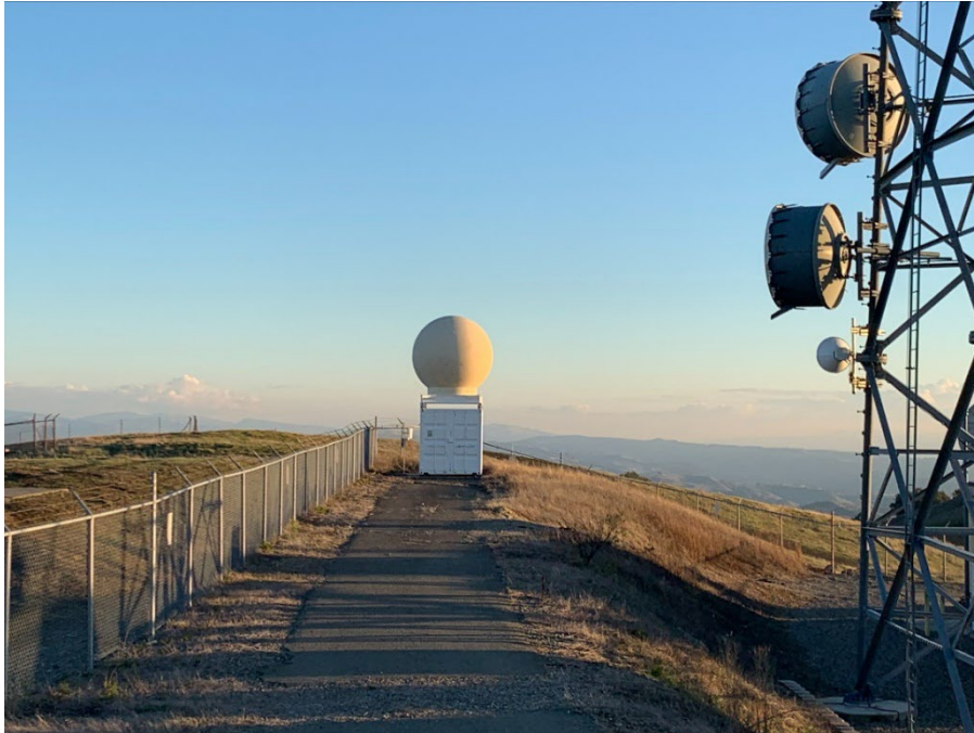
Figure 15. Rocky Ridge High Definition Doppler Radar Unit, December, 2022.
