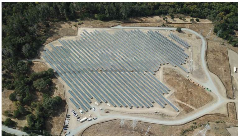
Figure 8. Duffel PV Project, October 2023.
