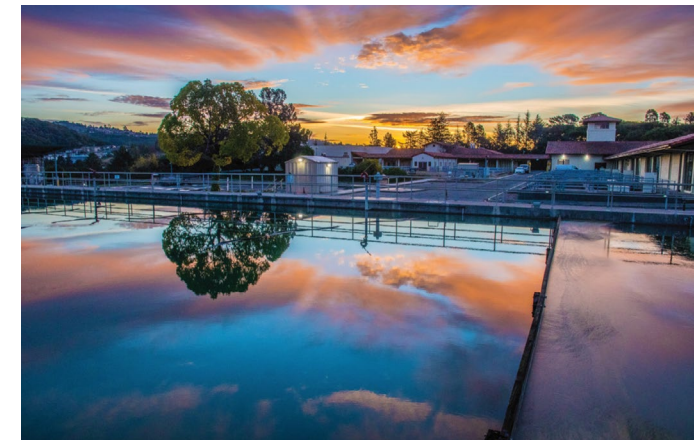
USL Water Treatment Plant.
