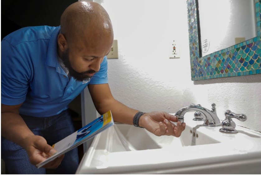
Figure 17. Installing an aerator on a bathroom faucet.
