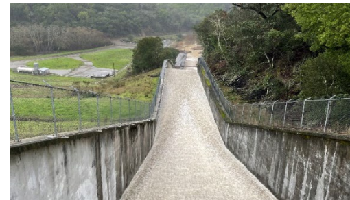
USL Reservoir Spillway
