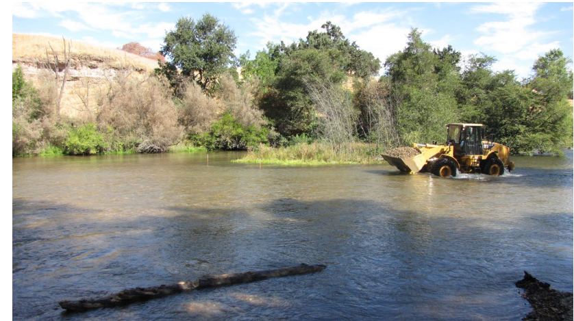
Gravel enhancement for spawning habitat on the Lower Mokelumne River.
