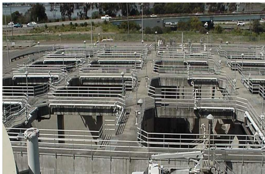
Wet Weather Flow Equalization Basin at the Main Wastewater Treatment Plant
