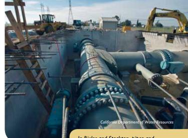
In Bixler and Stockton, pipes and valves have recently been installed between EBMUD's three aqueducts to connect them to each other. These interconnections will provide additional reliability in case one aqueduct is damaged in the Delta during an earthquake or flooding. The aqueducts deliver drinking water from the Sierra to East Bay homes, schools, fire hydrants and businesses.
