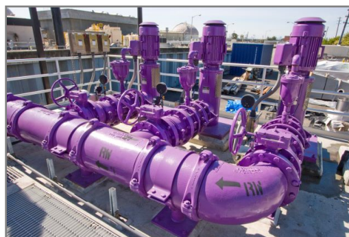
Recycled Water in Purple Pipes Provides an Important Source of Non-Potable Water
