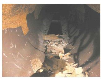
Delaminated lining accumulated on pipe invert
