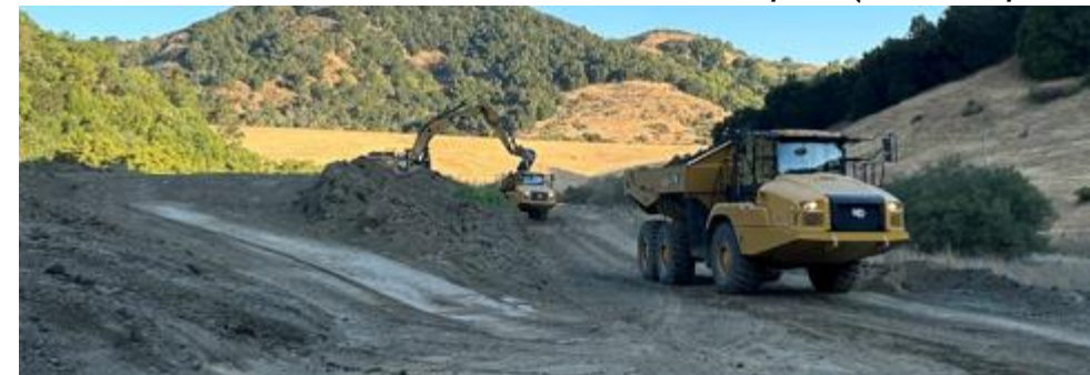
Loading Alameda County Landslide Repair Contractor Trucks
