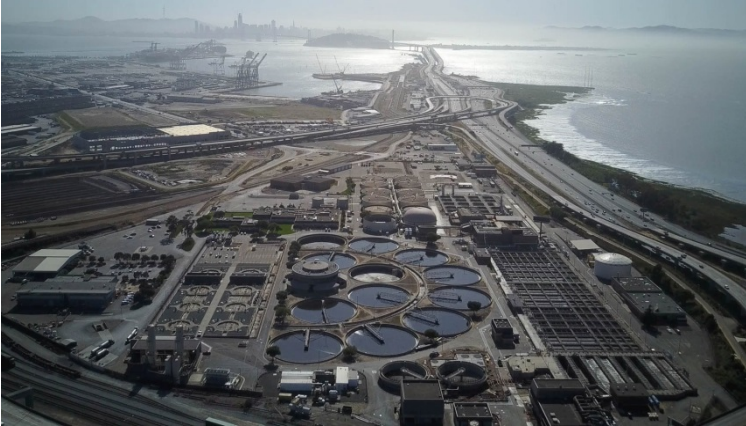
Wastewater Treatment Plant
