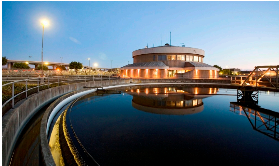
Main Wastewater Treatment Plant
