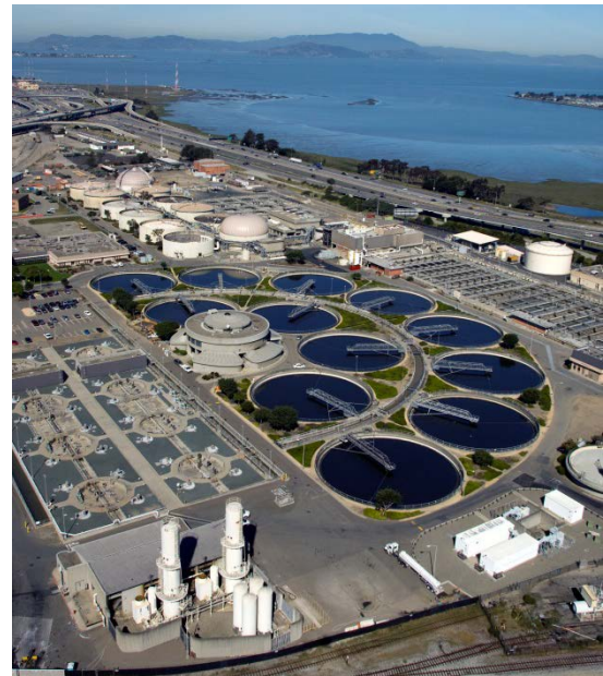
Wastewater Treatment Plant
