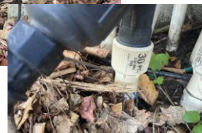
Drip pressure regulator and filter components
