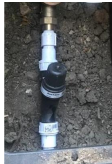
Drip pressure regulator and filter components
