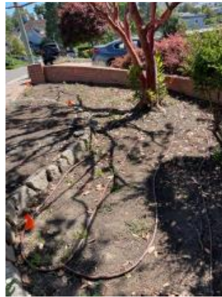
Drip tubing installed + mulch added
