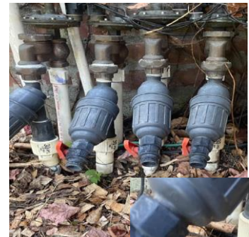
Drip pressure regulator and filter components
