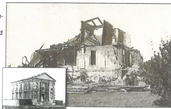
Figure 3. Photograph showing shaking damage from the 1868 magnitude-6.8 Hayward Fault earthquake, which caused collapse of the Alameda County Courthouse in San Leandro, California (photograph courtesy of the Bancroft Library, University of California, Berkeley). Inset shows the same building before the earthquake (photograph courtesy of San Leandro Public Library).
