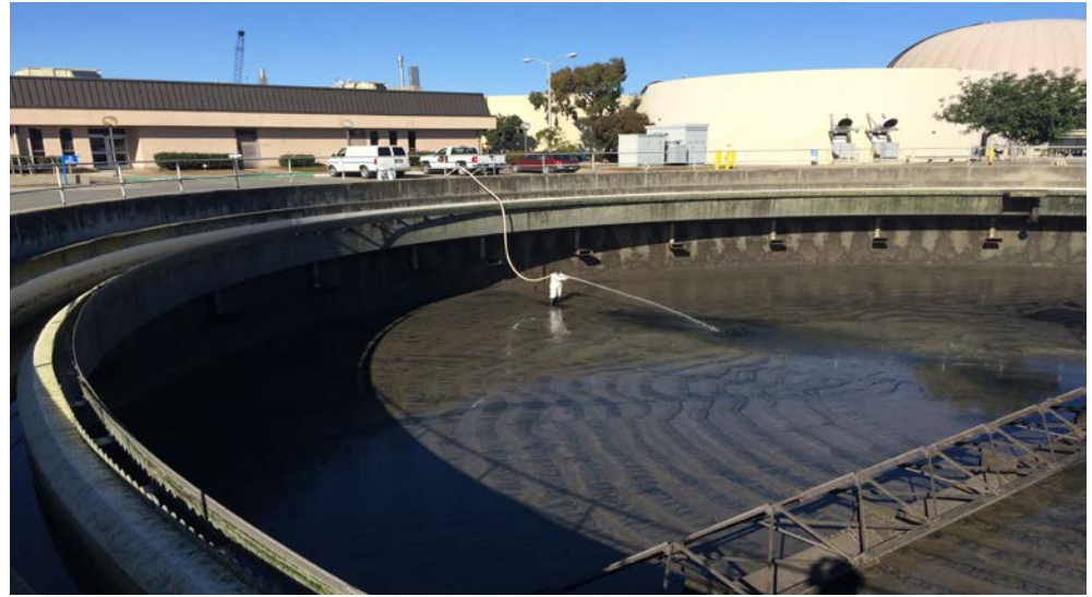
Flushing Solids from a Clarifier Being Taken Out of Service
