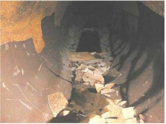
Delaminated lining accumulated on pipe invert
