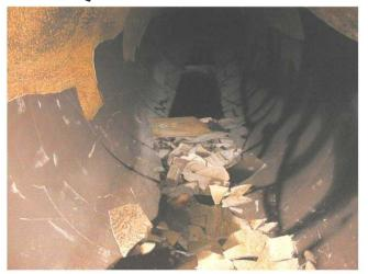
Delaminated lining accumulated on pipe invert
