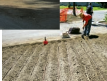
Below center: Sub-surface irrigation system is installed.
