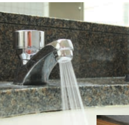
Above: Manual faucets in public restrooms provide adjustable timed water delivery.
