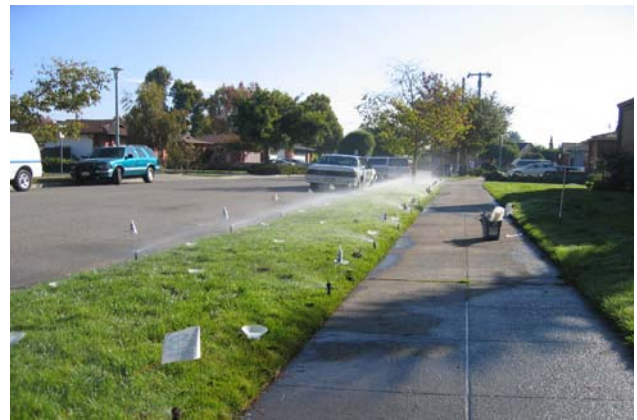
New sprinklers installed improved uniformity to 75%
