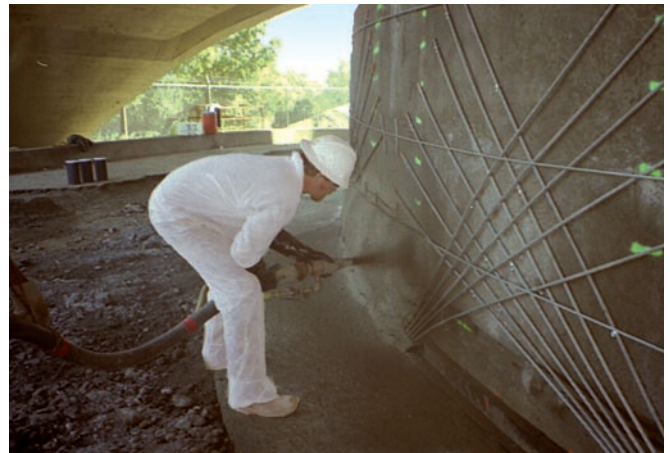
A reservoir is reinforced with seismic cables and shotcrete.
